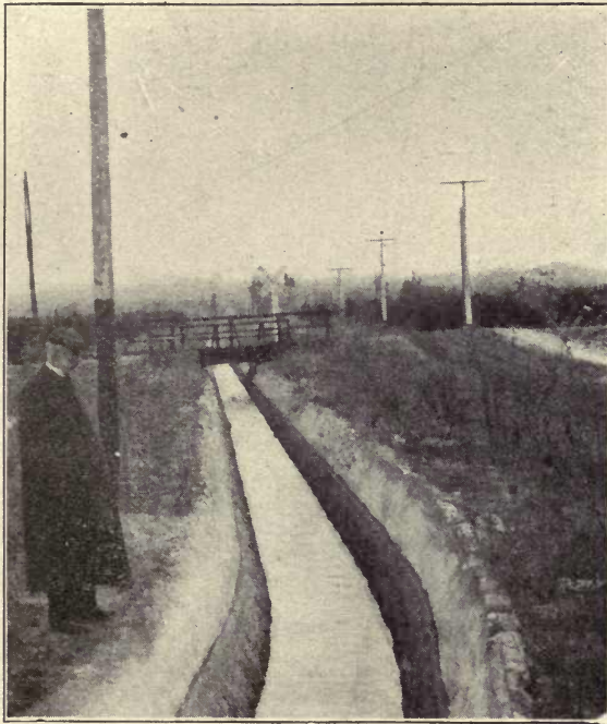
Fig. 149. Bear Valley Canal, Redlands, California. Boulder-lined and plastered.
