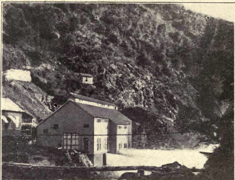
Fig. 190A. Exterior of Power-House, Showing Penstocks Delivering Water to Wheels under an Effective Head of 1,528 Feet.
