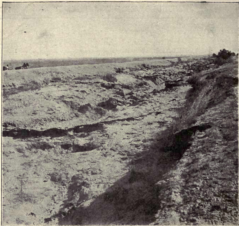
Fowler Switch Canal, California, Showing Effect of High Velocities.
