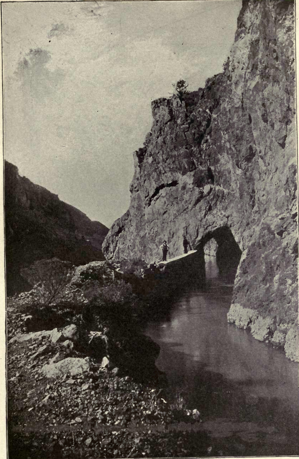
Fig. 151. Tunnel of Bear River Canal, Utah.
