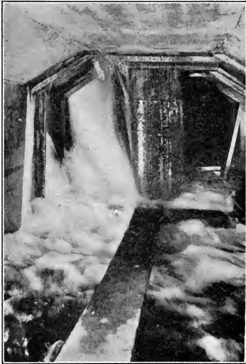
FIG. 180.—Discharge from relief valve when opened.
