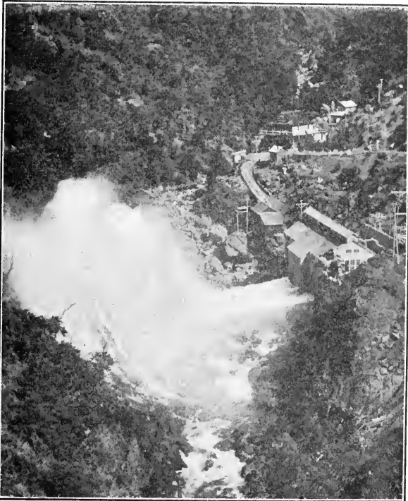
From a photograph by F. H. Fowler. FIG. 164.—DeSabra power plant with nozzles deflected.
