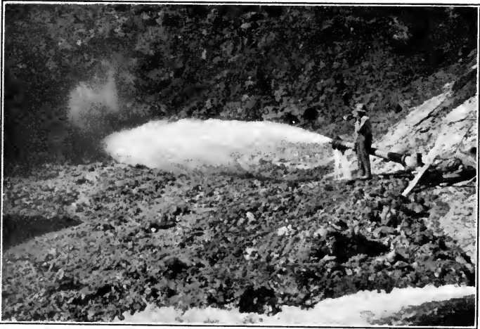
FIG. 66.—Jet from hydraulic giant sluicing out material for Calaveras earth dam.
