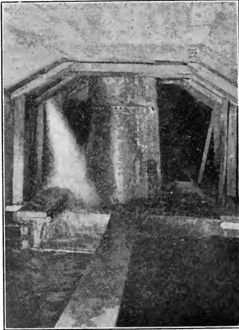
FIG. 179.—Small discharge from relief valve near draft tube in Cornell University power plant.
