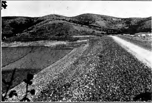
FIG. 37.—Upstream face of San Andreas earth dam. 90 ft. high.
