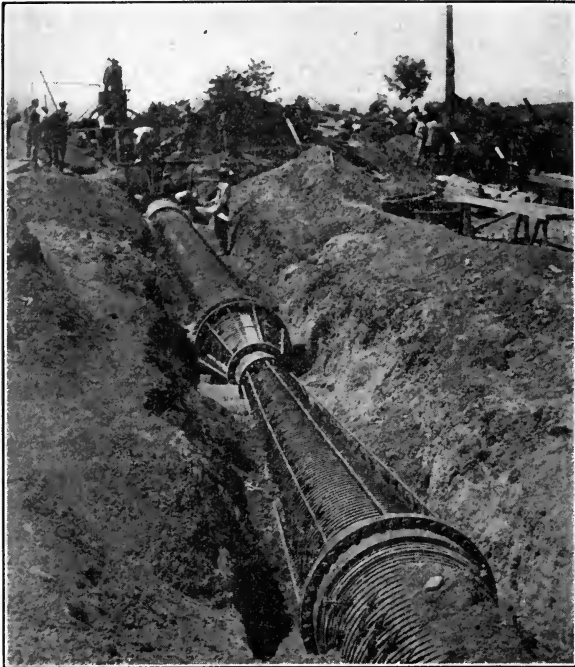
FIG. 77.—Venturi meter in wood pipe line.
