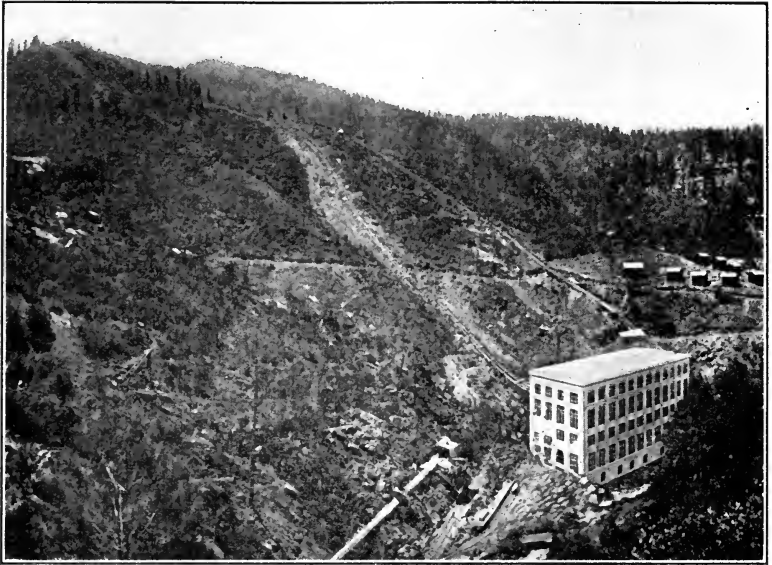
FIG. 199.—Power Plant No. 2 at Big Creek. Static head = 1900 ft.; Hp. = 40,000.
