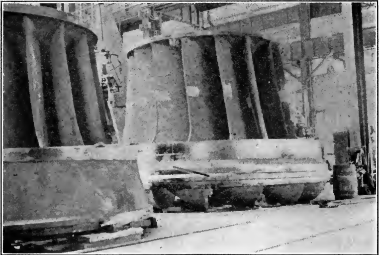
FIG. 170.—The largest turbine runner in the world. For Cedars Rapids Mfg. and Power Co. D = 143'' ; h = 30' ; N = 55.6 ; Hp = 10,800 .
