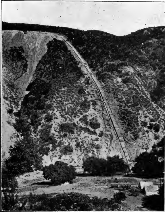
FIG. 126.—Open channel with steep slope. Future power site on Los Angeles Aqueduct. Drop in elevation = 524 ft.
