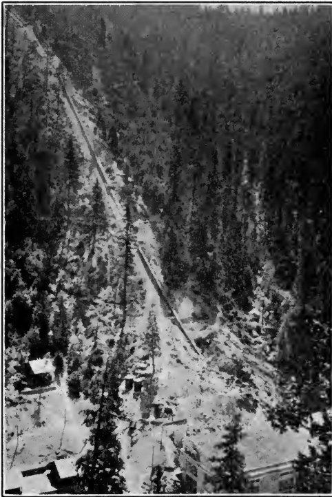
FIG. 191.—Penstock leading to Drum power house of Pacific Gas & Elec. Co. under 1375 ft. head.
