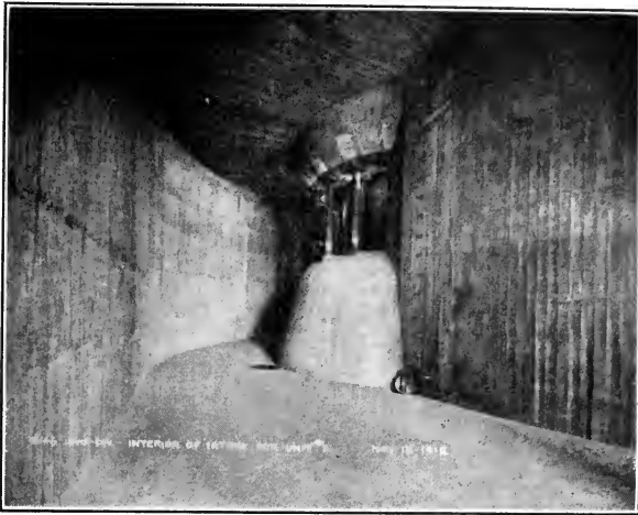
FIG. 187.—Intake for turbine at Keokuk.
