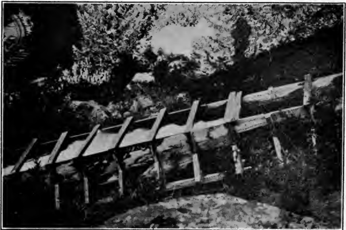
FIG. 123.—Non-uniform flow in wooden flume.
