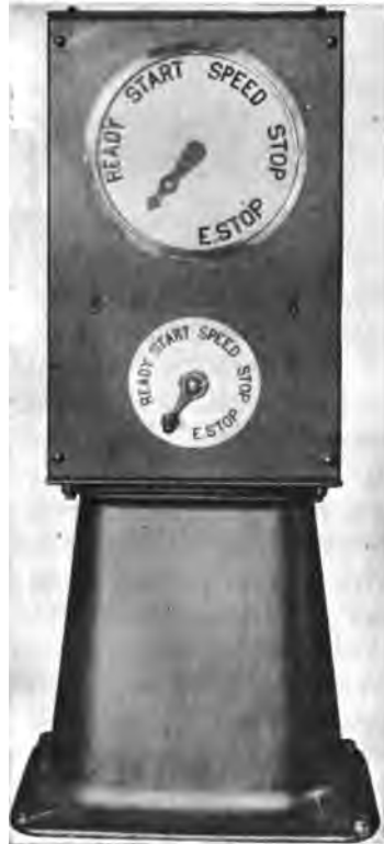
FIG. 378.—Signal Equipment at Mississippi River Power Company. Generator Room Pedestal.
