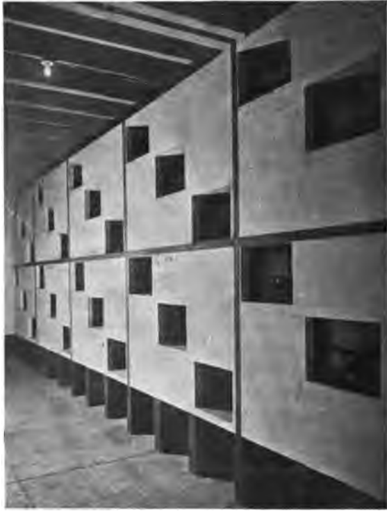
FIG. 363.—Low-tension Bus Compartments.
