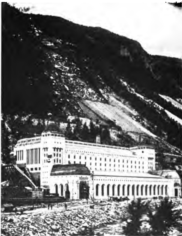
FIG. 9.—Rjukan II Power and Furnace House for Nitrogen Fixation in Norway. Capacity 120,000 horse-power.
