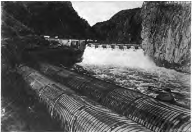
FIG. 65.—Montana Power Company. Dam and Wooden Penstocks for Madison No. 2 Plant.
