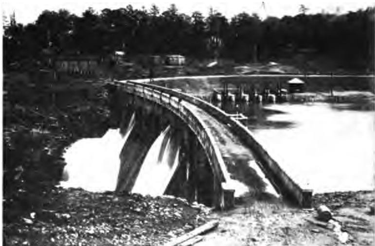
FIG. 51.—Tunnel Intake, Showing Its Relation to the Diversion Dam.
