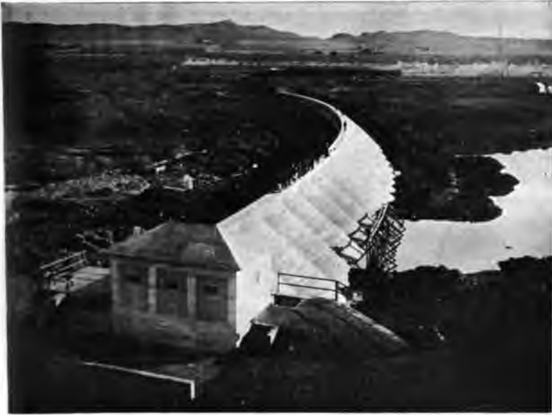
FIG. 41.—Multiple-Arched Dam. Umatilla Project, Oregon.
