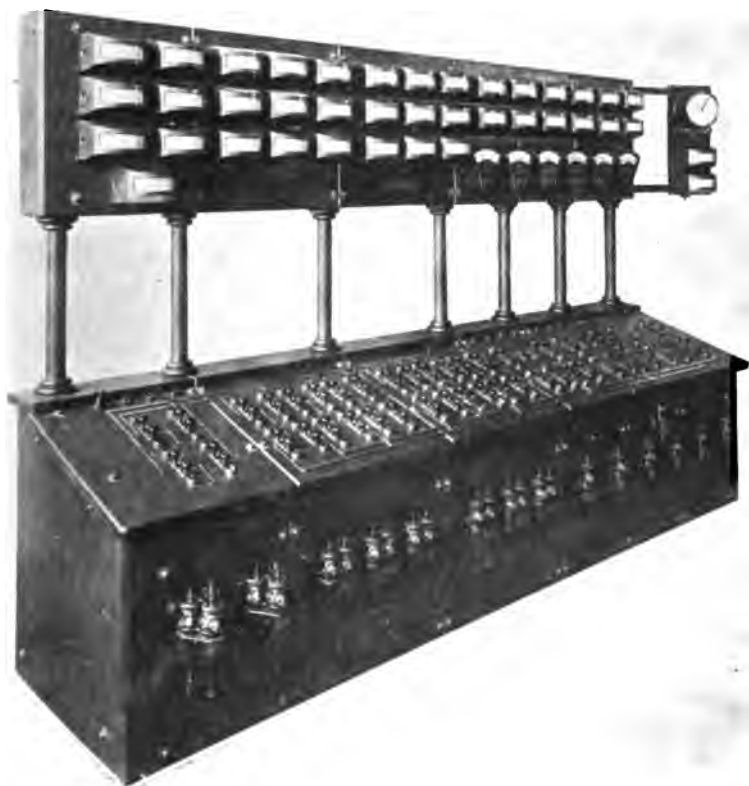
FIG. 343.—Typical Benchboard of the Gallery Type.
