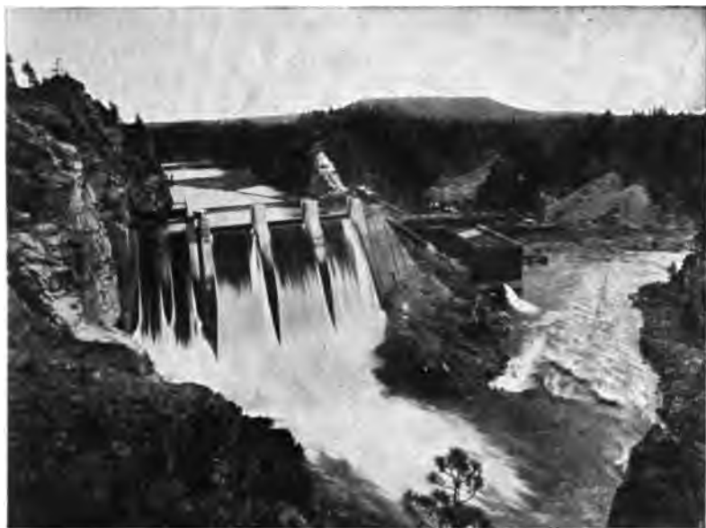
FIG. 49A.—Dam of Wasnington Water Power Company, Showing Arrangement of Rolling Gates.
