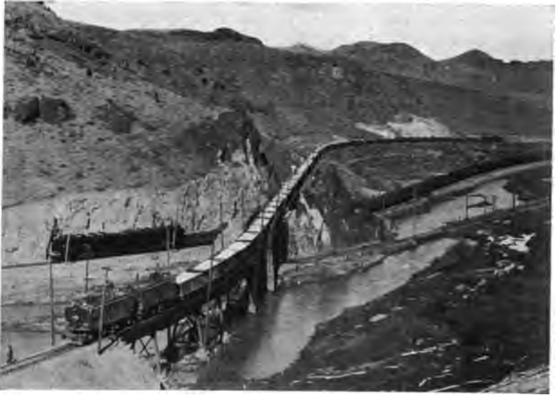
FIG. 10.—Electric Trains at the Entrance to Silver Bow Canyon on the Chicago, Milwaukee & St. Paul and the Butte, Anaconda & Pacific Railways.
