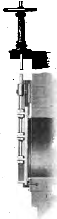
FIG. 72.—Rising Stem Sluice Gate. Side View of Gate Shown in Fig. 71.
