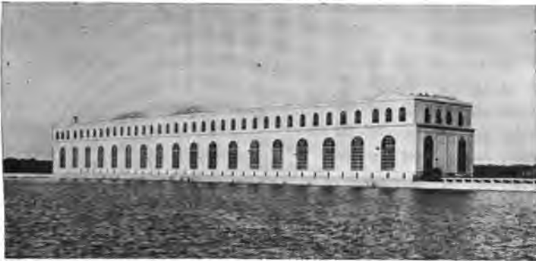
FIG. 87.—Power House, Mississippi River Power Company, Keokuk, Iowa.
