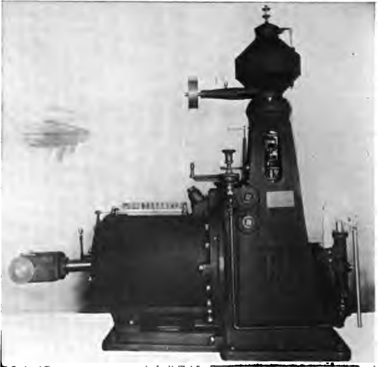
FIG. 137.—Lombard Type T Governor.
