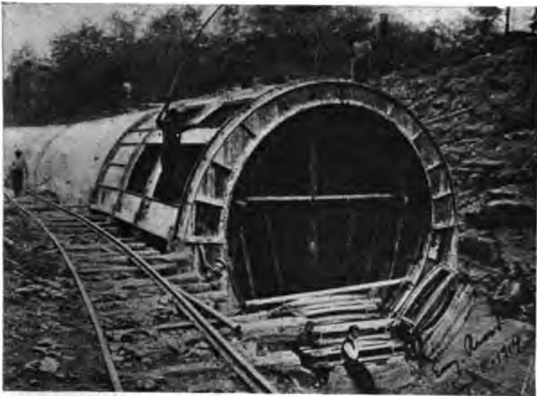
FIG. 66.—Concrete Pipe, Showing Steel Forms for Pouring.
