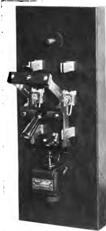
FIG. 350.—Automatic Throw-over Switch.
