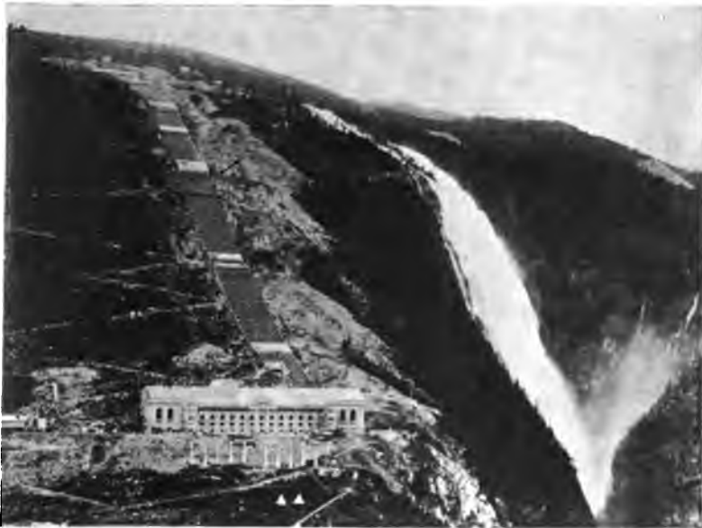
FIG. 62.—Large Hydro-Electric Power Station at Rjukan, Norway, Showing Ten Five-foot Penstocks and Method of Anchoring Same.
