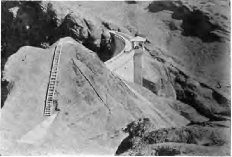
FIG. 39.—Arched Dam. Orland Project, California.
