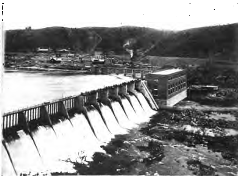
FIG. 36.—Typical Masonry Dam of the Gravity Type. Appalachian Power Company.
