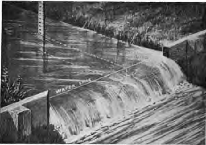
FIG. 19.—Weir for Measuring Flow of Water.
