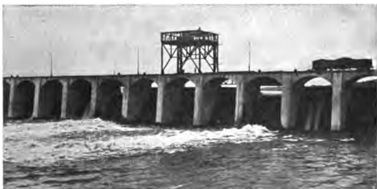
FIG. 44.—Spillway Gates. Mississippi River Power Company, Keokuk, Iowa.
