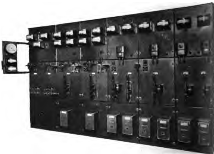
FIG. 335.—Typical Vertical-type Switchboard with Hand-operated Oil Circuit Breakers. Front View.
