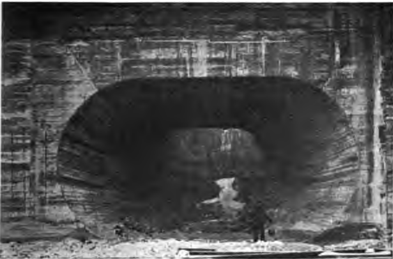
FIG. 132.—Lower End of a Molded Concrete Draft Tube.
