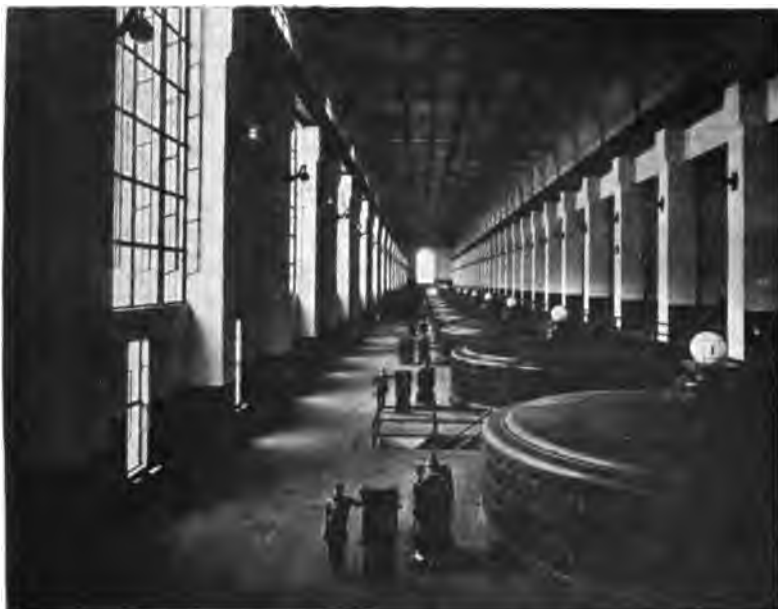
FIG. 3.—Power House, Mississippi River Power Company, Keokuk, Iowa.
