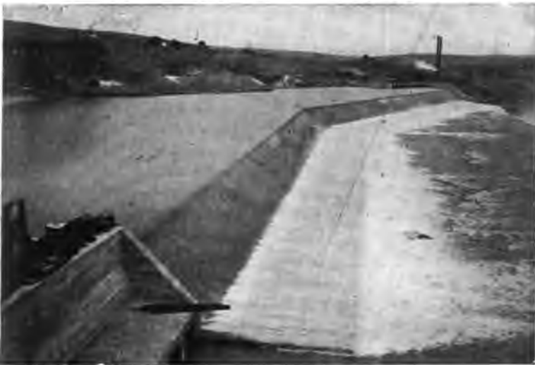
FIG. 28.—Timber Crib Dam, Montana Power Company.
