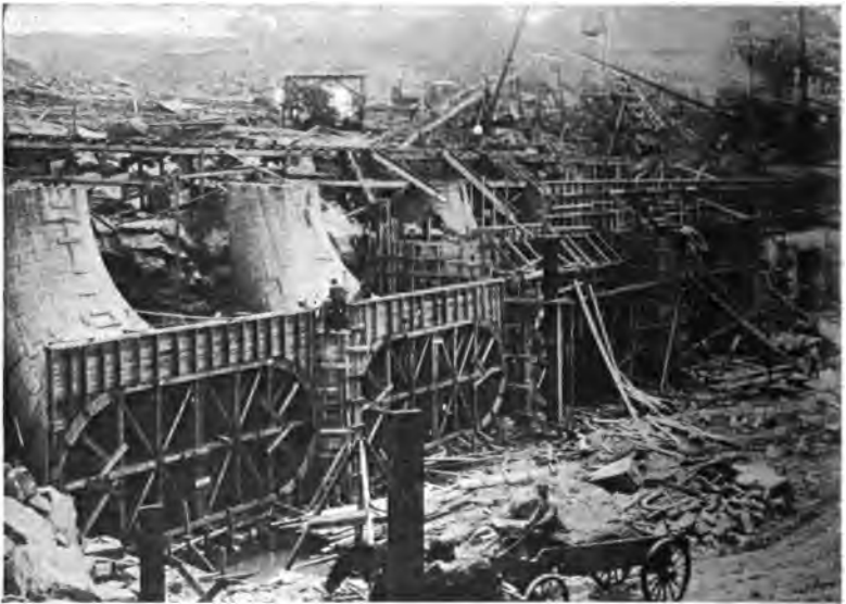
FIG. 131.—Placing of Wooden Forms for Draft Tubes of Three 10,000 Horsepower Turbines.
