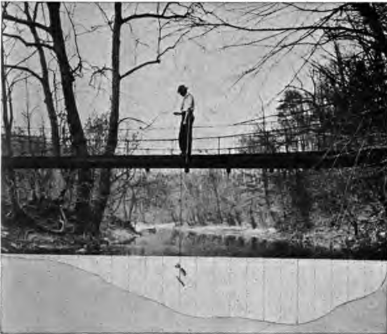
FIG. 22.—Typical Gauging Station for Bridge Measurement.
