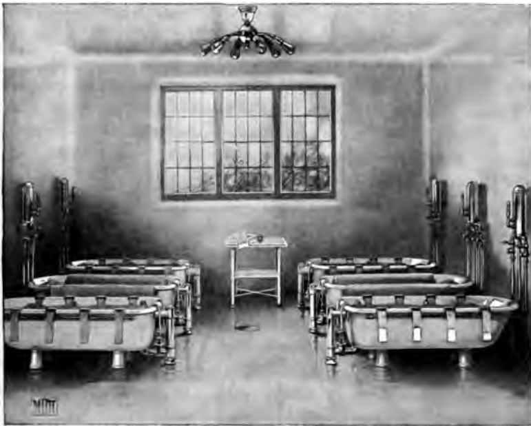
Fig. 85.—Interior of room for continuous baths (J. L. Mott Iron Works).
