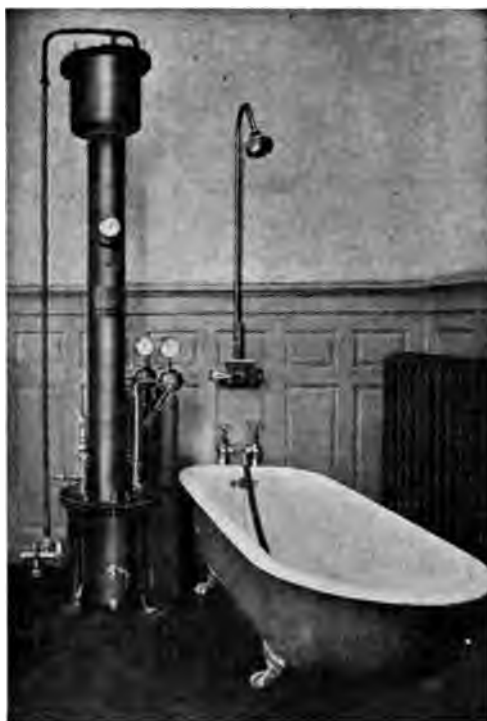
Fig. 101.—The Fischer-Kiefer CO 2 generator for Nauheim bath (Luke).
