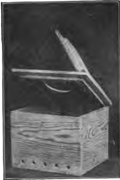
FIG. 35.—PRIVY BOX OF ONE-CAN ADJUSTABLE COVER TYPE.
