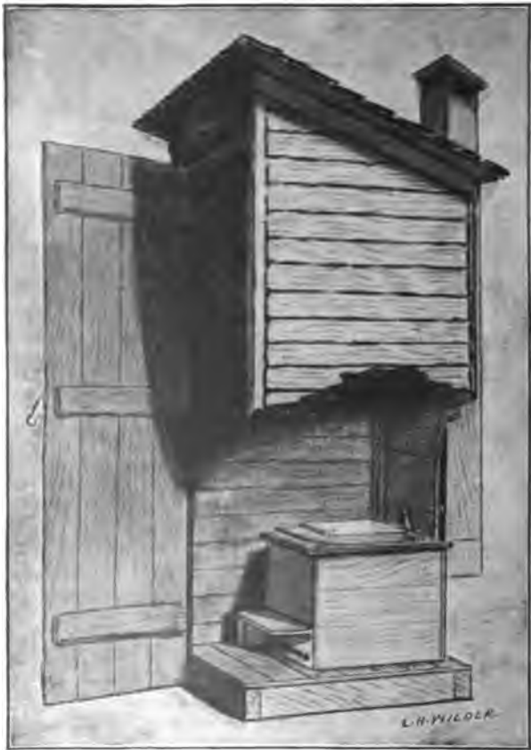
FIG. 33.—ONE-CAN ADJUSTABLE-COVER AND VENT-FLUE INSTALLED IN PRIVY. ( Public Health Bulletin, No. 89. )
