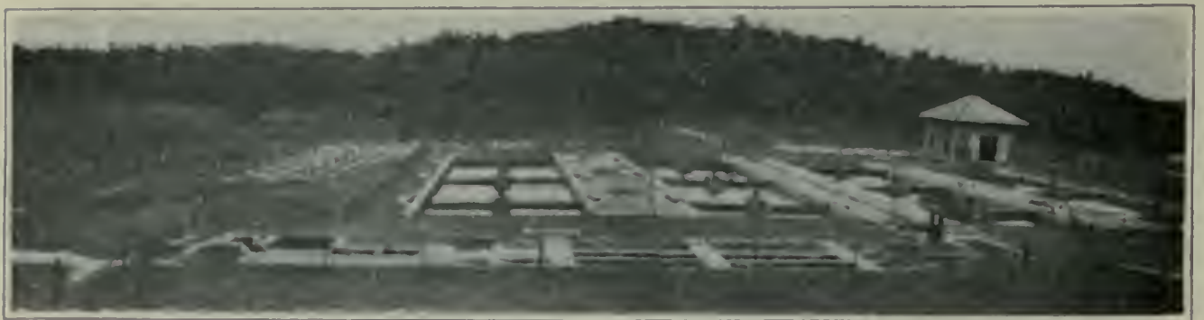
Fig. 41.—Sewage purification plant at Atlanta, Ga. In the foreground there are grit chambers in which the sand is settled out. The water then flows into the large Imhoff Tanks beyond and from these tanks the effluent is carried to trickling filters some of which are seen in action. To the extreme left a sand bed for drying the sludge appears in indistinct outline.
