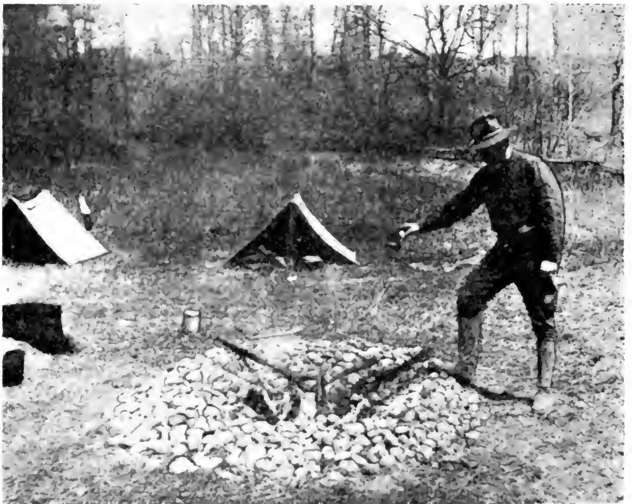
Fig. 44.— Outdoor incinerator (Arnold type). (Gardner.)
