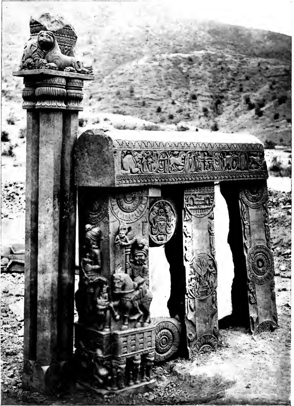
THE BHARHUT RAIL : EAST GATEWAY
