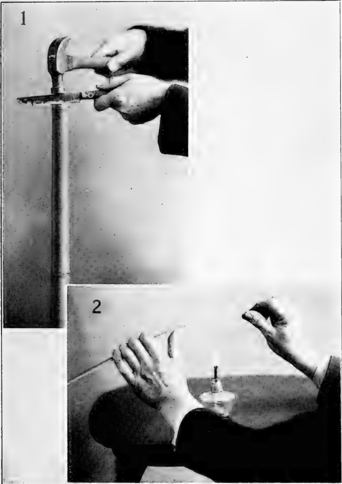
1—Halving stalks 2—Corrective bending over alcohol lamp
