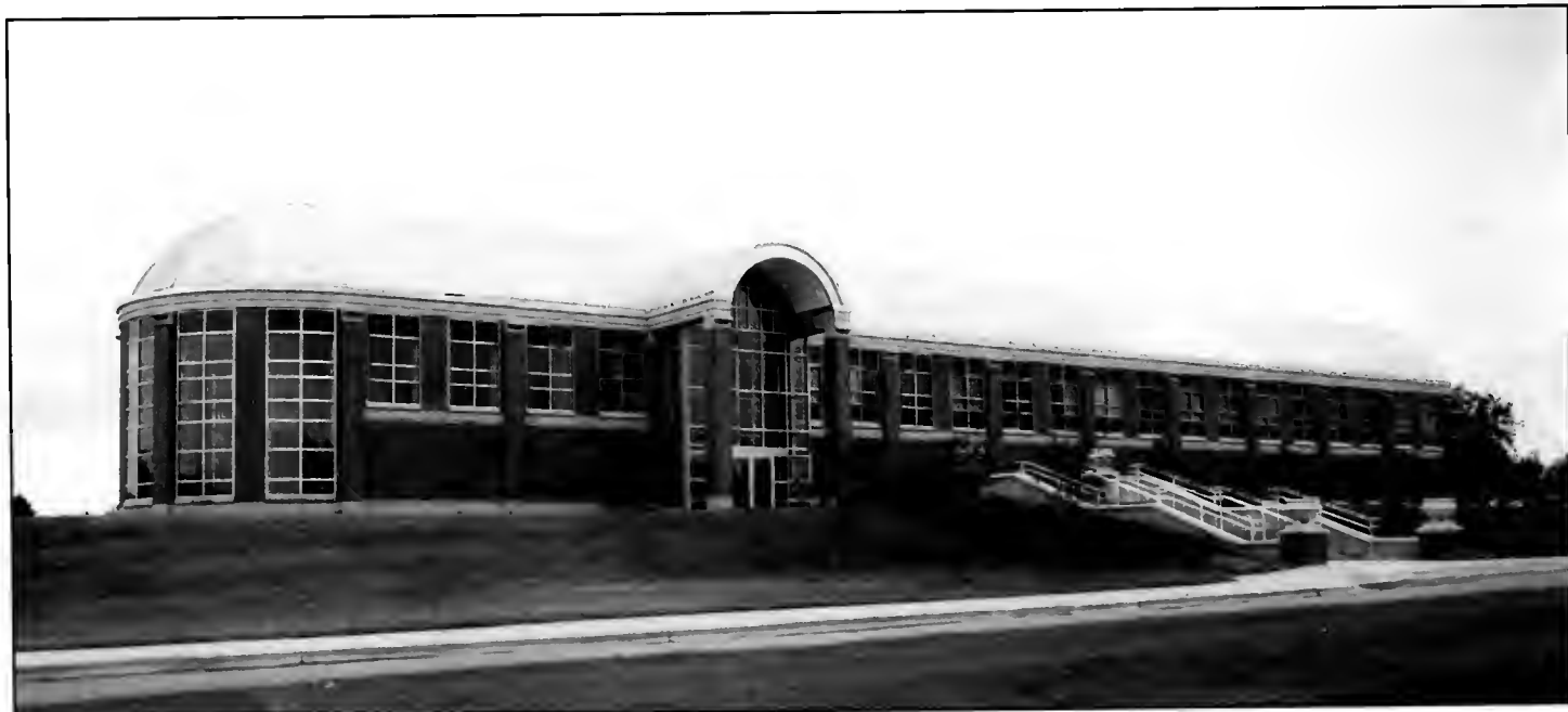
The Bielfeldt Athletic Administration Building houses coaches and administration for the Division of Intercollegiate Athletics.
