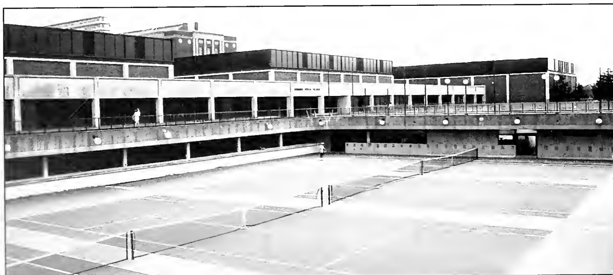
The Intramural and Physical Education Building is one of the largest complexes of its type on any college campus.
