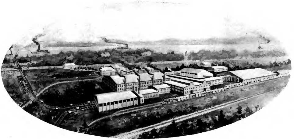
CEMENT PLANT, KOSMOSDALE, KY., NEAR LOUISVILLE.
