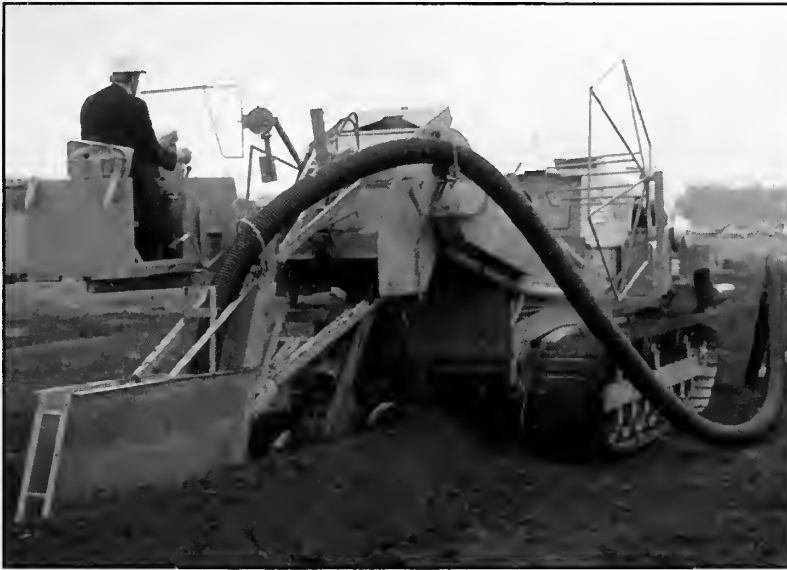
Installing drainage tile. Drainage tile is used extensively in central Illinois to remove excess water from farmland.
