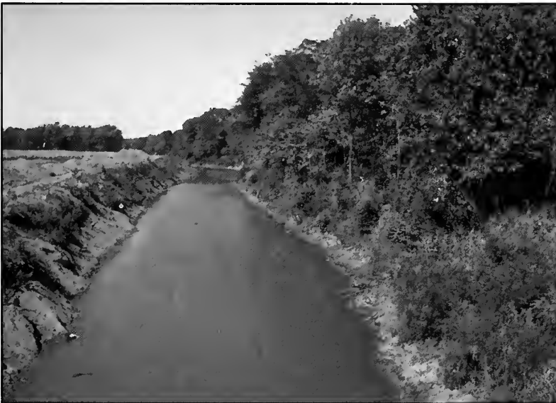
Balancing drainage and environmental considerations. This drainage ditch remains clear on one side. The trees that have been allowed to grow on the other side provide a habitat for wildlife.
