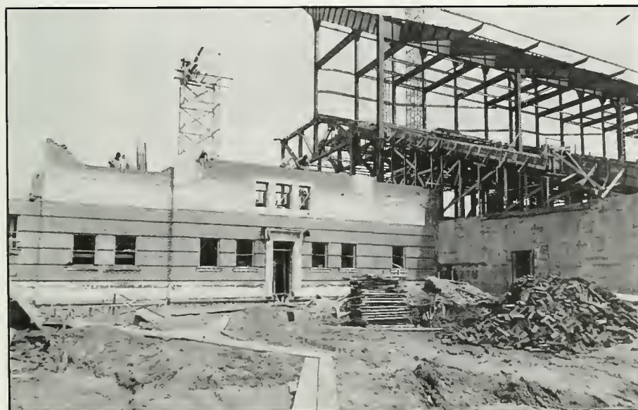
Memorial Stadium was constructed in 1923 and was funded by $1.7 million in donations from University students, alumni and friends.
