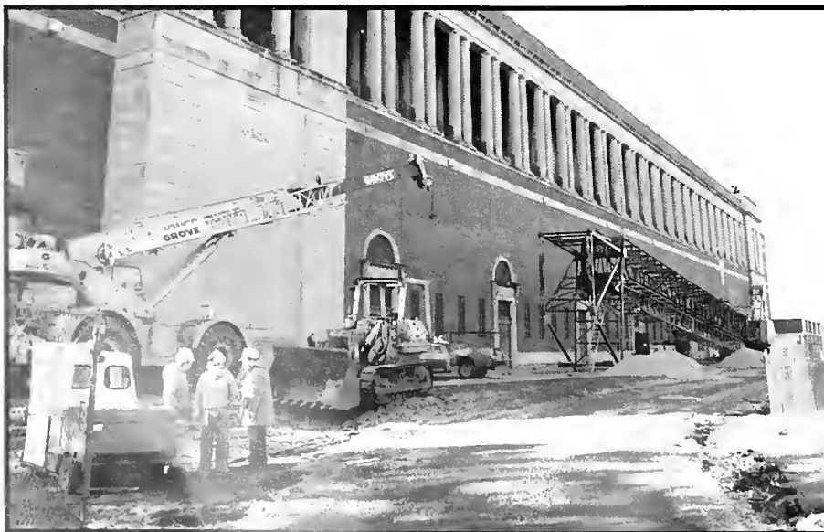
From November 1991 until August 1992, Memorial Stadium underwent an $18 million renovation.
