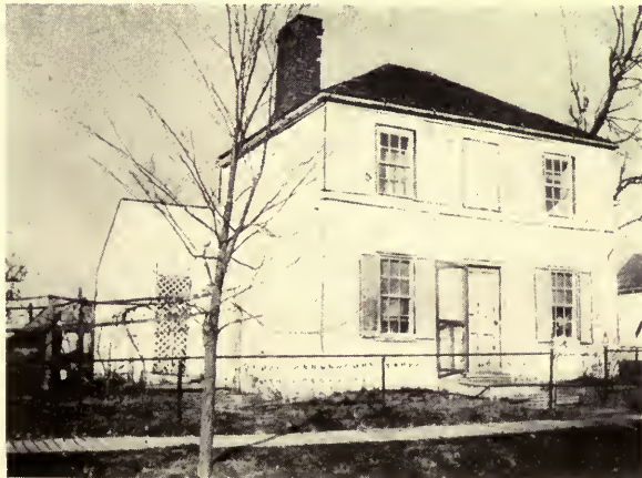
COTTAGE AT ALBION, BUILT NINETY-FIVE YEARS AGO, OCCUPIED CONTINUOUSLY, AND STILL STANDING
