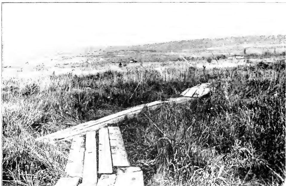
THE BEGINNING OF ONE OF THE PASSERALLES ACROSS FORGES SWAMP
