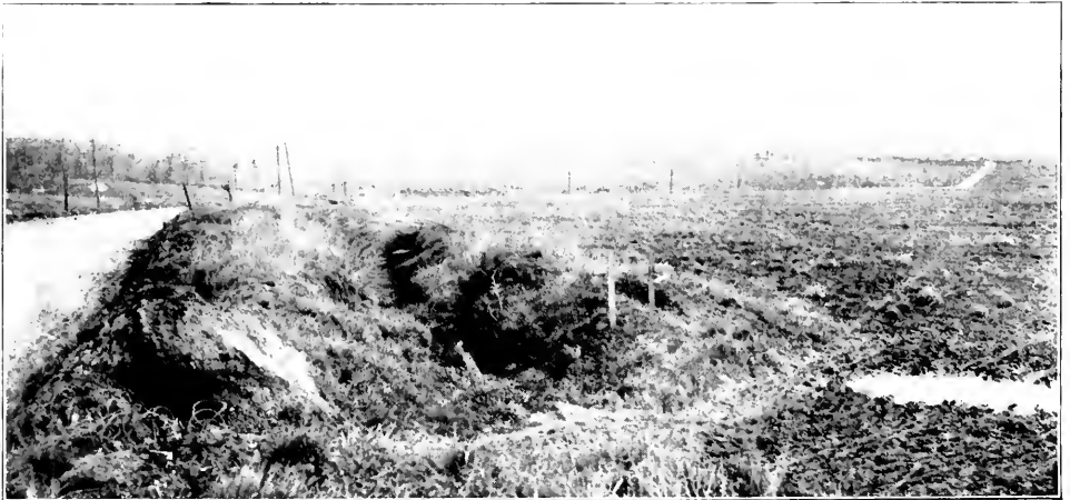
TRENCHES ALONG THE BRAY-CORBIE ROAD HELD BY THE 131ST INFANTRY ON THE MORNING OF AUGUST 10.
