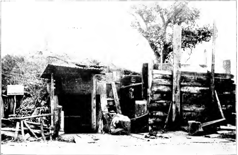
GERMAN ELECTRIC POWER PLANT AT GERCOURT
