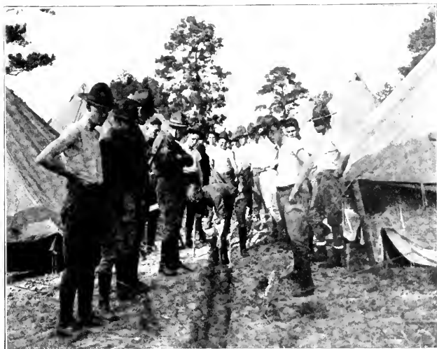
AND SOME DUG DITCHES
