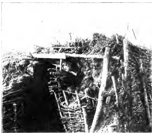
TYPICAL REVETMENTS ON THE ROAD TO XIVRAY
