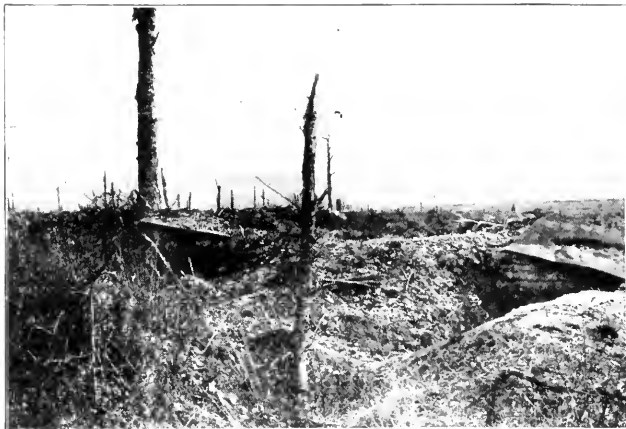
GERMAN OBSERVATION POST IN CERVAUX TRENCH
