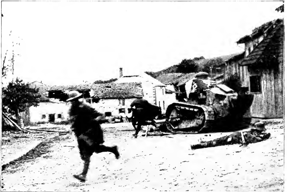
A DANGEROUS CORNER IN EXERMONT
