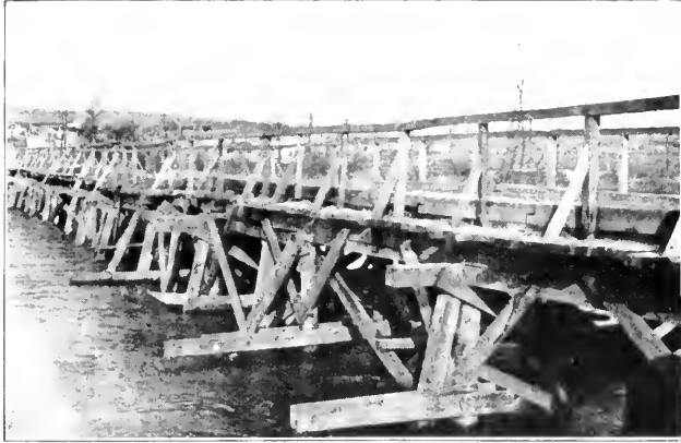
THE WORK OF THE 108TH ENGINEERS One of the bridges over the Meuse at Consenvoye.
