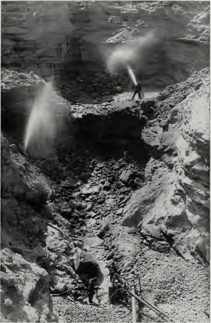
Hydraulic mining of silica sand in LaSalle County
