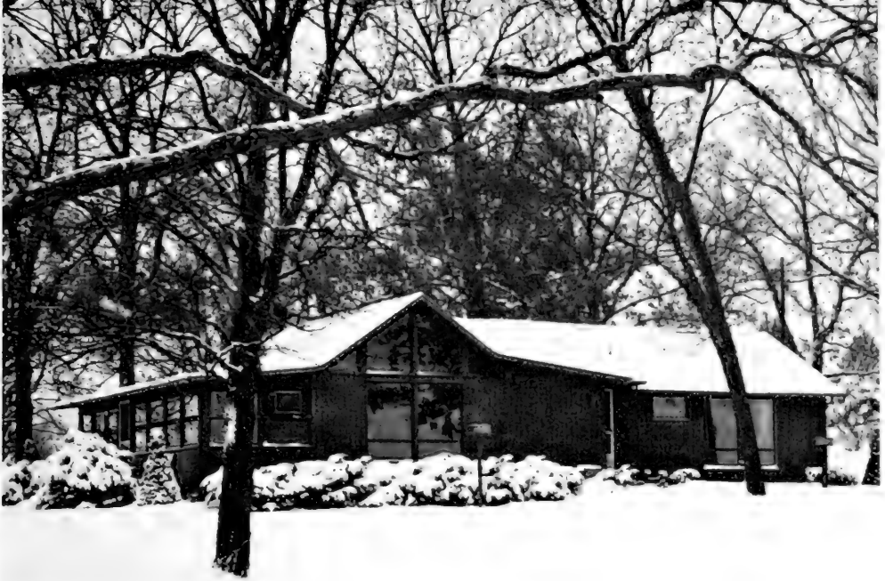
Newly converted Survey field station designed for studies on the biology of the Kaskaskia River and Lake Shelbyville. (Photo by Warren Brigham.)
