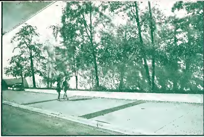
Trees improve the appearance of this industrial building, but may be planted too close to it to allow for maximum growth.
