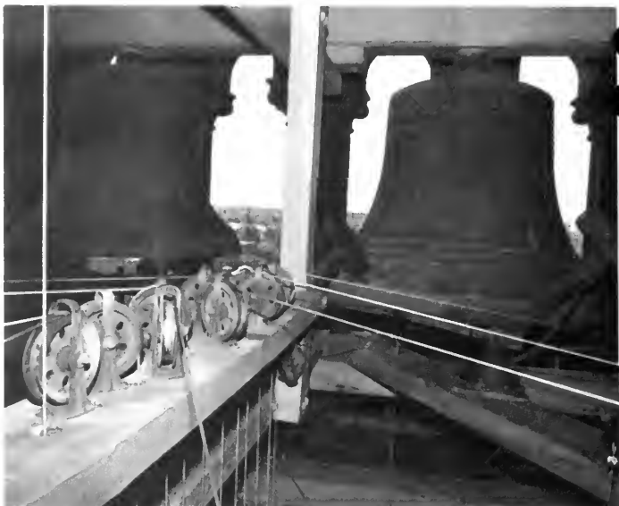
The familiar ringing of the Altgeld chimes is accomplished with a hammer and clapper system as seen on the left. Seen above is the aircraft cable and pulley system used for moving the clapper (photos by Mike Brooks).
