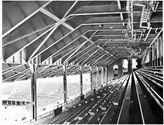
After extensive fundraising, construction began on Memorial Stadium in 1922. Ramps, gutters, and an upper deck were among the unusual attributes of the new facility. (Daily Illini file photo)
