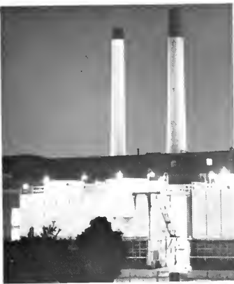
Abbott power plant provides the University with its primary source of electricity and steam. Constructed in 1941, the plant continually improves its safety and efficiency. (Photo by Dave Colburn)
