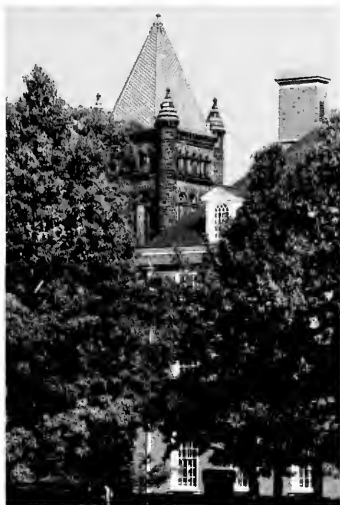
Algeld Hall was originally constructed as the University's library in 1897, while the Illini Union was constructed on the site of University Hall in 1941. (Photo by Phil Messersmith)
