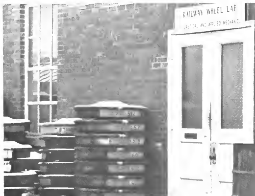
Constructed in 1912, the Railway Wheel Lab played a major role in exploring improved methods and machinery for the railroading industry. Although the importance of rail transportation has since waned, research on the possibilities for today's rail industry still plays an important role at the University. (Photo by Mike Brooks)
