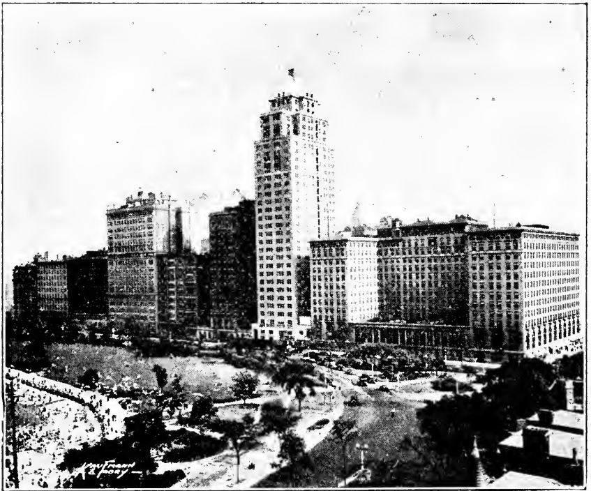
View looking south from Lake Shore Drive, showing prominent apartment buildings, the Drake Tower and the Drake Hotel at the extreme right. In the left foreground are Oak Street Beach and the Park, which make this a particularly attractive spot for tourists.
