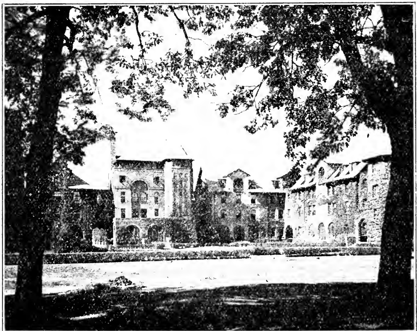
Fraternity houses and men's dormitories on campus of Northwestern University, Evanston. Dr. Walter Dill Scott is president.
