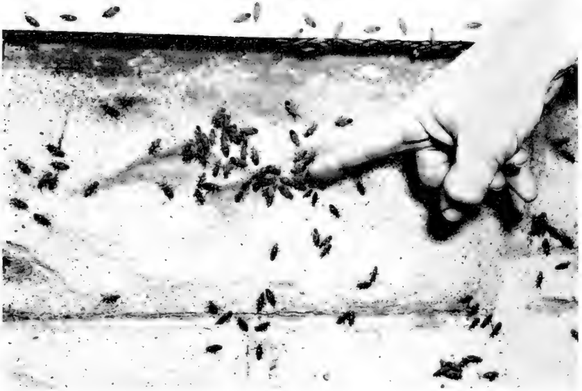
Fig. 7.—Boxelder bug: adults. Shown here are boxelder bugs on the foundation of a building. The bugs, which are black and red in color, are of no consequence as pests of boxelder trees, but they are nuisances in and on buildings.
