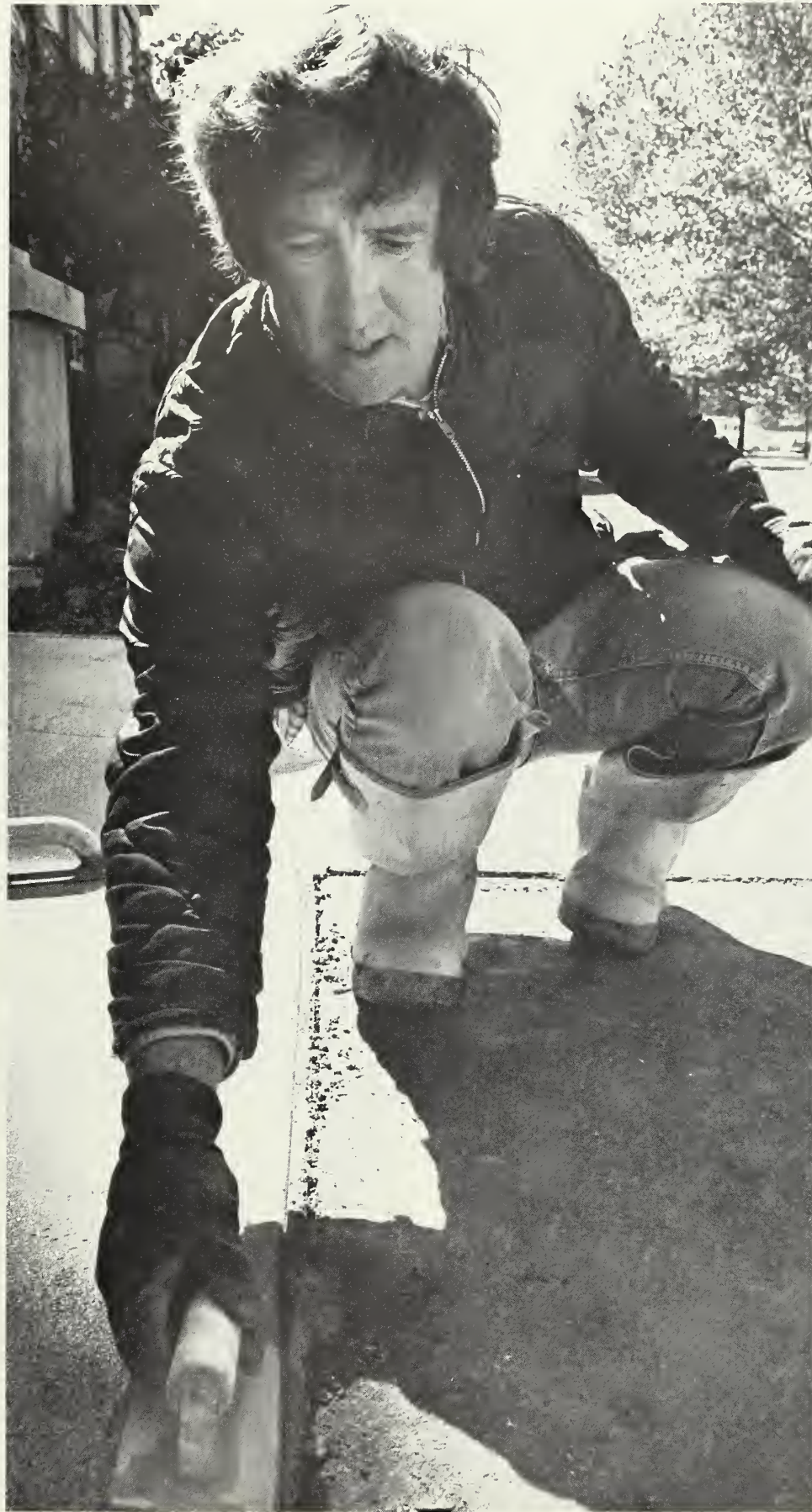
Ronald Eades, part of one of the many construction crews on campus, edges cement for new sidewalks near Mumford Hall.
