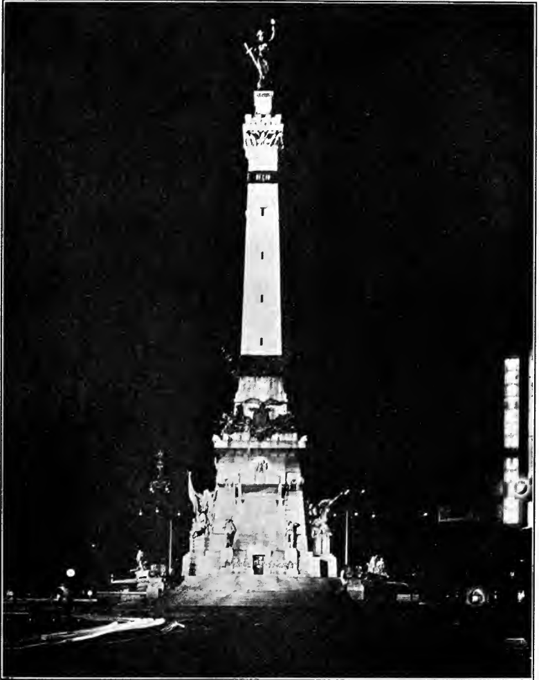
Fig. 31.—Representative flood-lighting installation.
