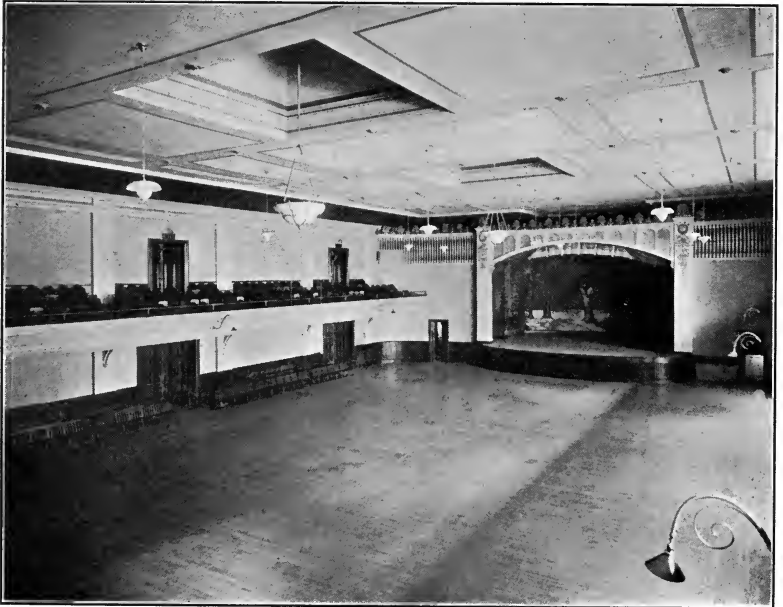
Fig. 21.—2000-c.p. fixtures installed. (The small fixtures belong to the previous installation.)
