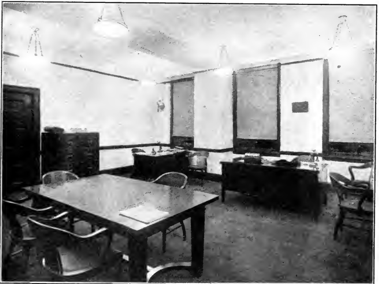
Fig. 2.—Medium-size private office. Ceiling height 10.5 ft. Ceiling finish white, walls dark cream. Six outlets are used with three 60-watt clear tungsten lamps in semi-indirect dishes at each outlet. Length of fixture 2.5 ft.
