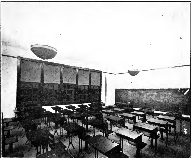
Fig. 8.—Classroom lighting with a few indirect units.
