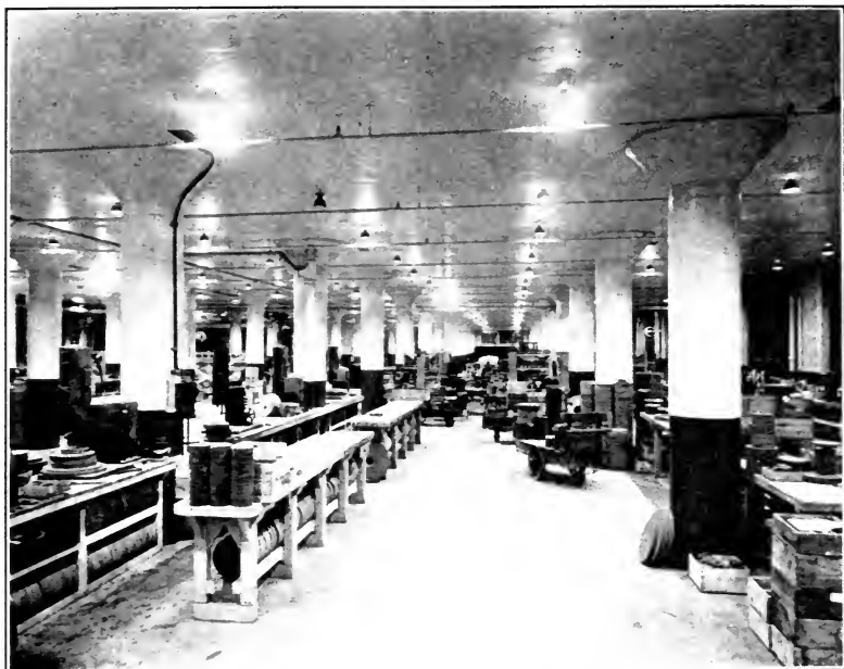
Fig. 1.—Tungsten direct lighting with opaque mirrored glass reflectors.
