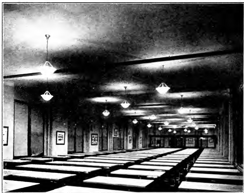
Fig. 2.—Drafting room with a system of semi-indirect tungsten lighting.
