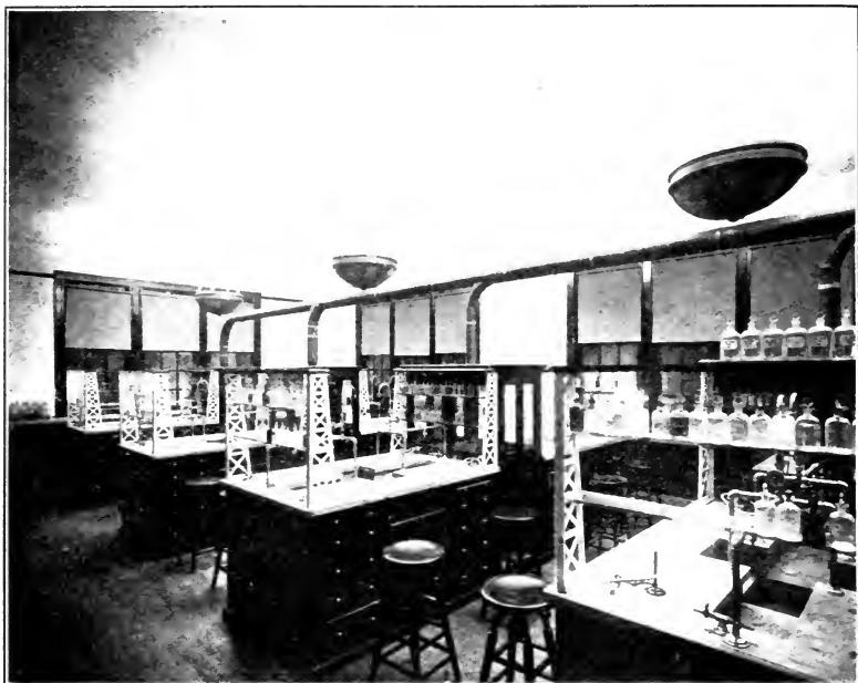
Fig. 5.—Indirect lighting of chemical laboratory.
