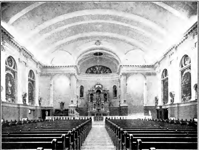
Fig. 8.—Ritualistic church. A good example of indirect lighting by means of lamps concealed on top of cornice.
