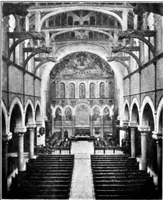
Fig. 4.—Evangelical church. Good example of semi-concealed lighting. Lamps, with proper reflectors, are placed on the chancel side of the hammer beams and in the rear of the chancel.
