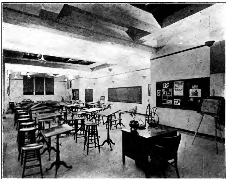
Fig. 2.—A drawing room properly illuminated by a totally indirect system, with simple opaque fixtures.
