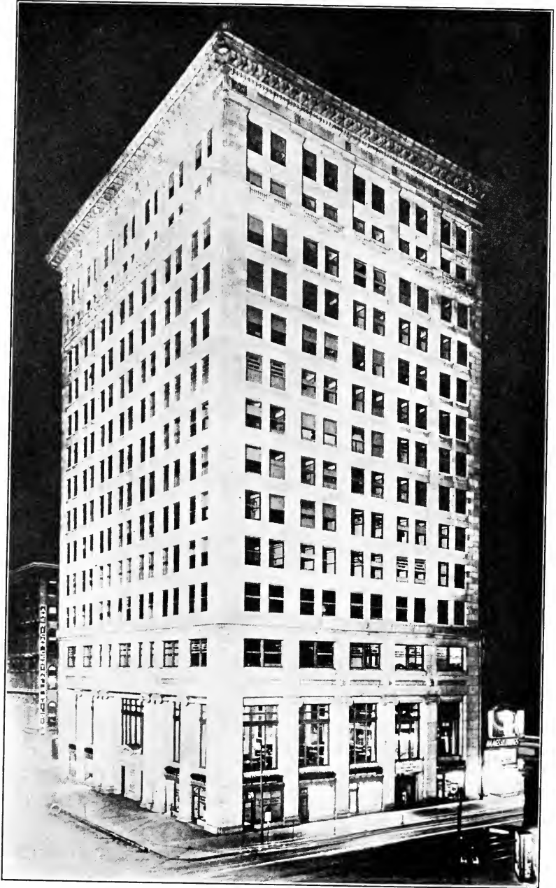
Fig. 28.—Representative flood-lighting installation.
