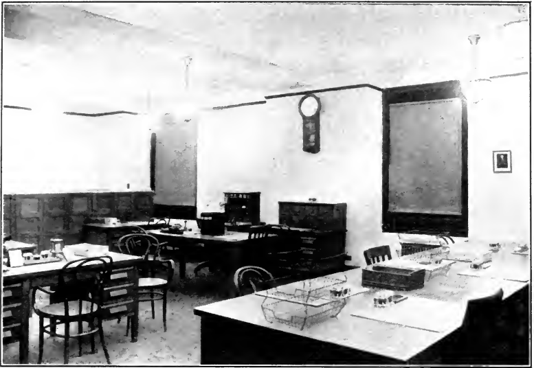
Fig. 1.—Office 30 ft. by 32 ft., ceiling height 10 ft. 6 in. Ceiling is matt white in color, walls medium cream. Height to bottom of units 8 ft. Seven semi-indirect lighting fixtures are used with dense opal glass reflectors. One 300-watt gas-filled lamp per outlet.
