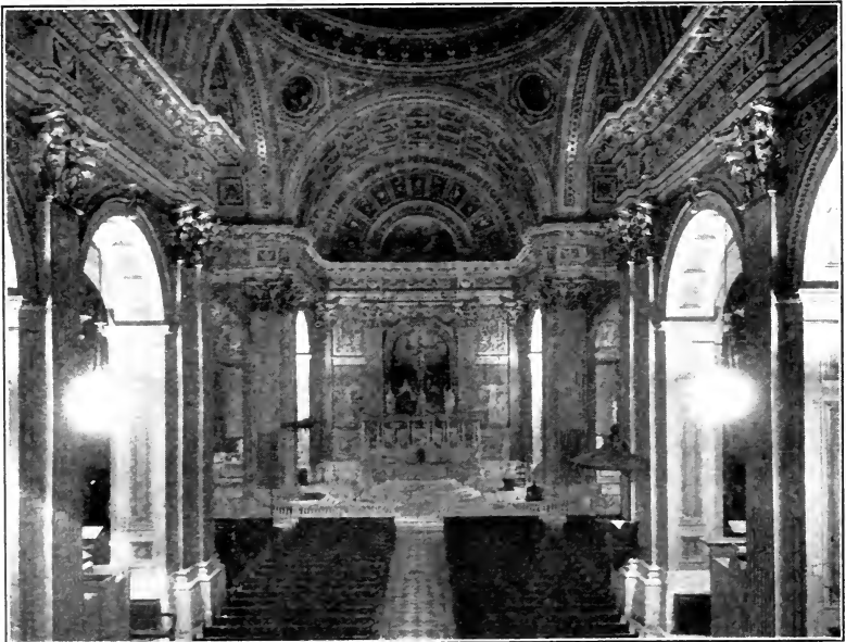
Fig. 10.—R. C. cathedral of Philadelphia. Semi-indirect lighting illustrating the diffusion obtained by the improved method of installation.
