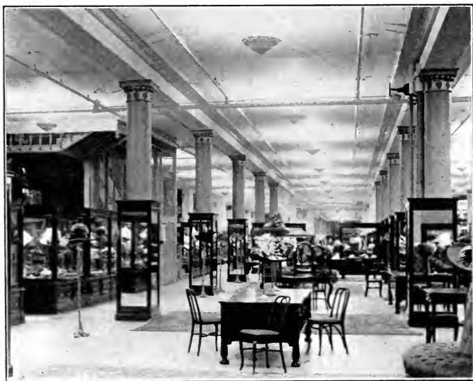
Fig. 6.—View of floor of large department store using enamelled steel indirect lighting fixtures with short suspension. A better distribution of light could be secured in this kind of location if the fixtures were lower so that the ceiling would be more uniformly lighted.
