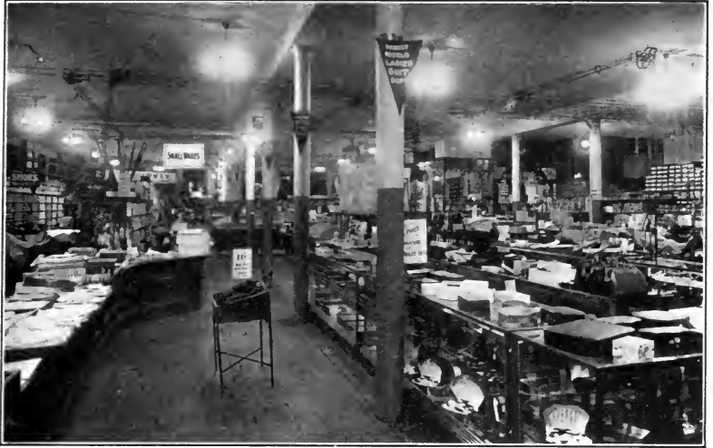
Fig. 9.—Small department store using three-lamp fixtures with single inverted mantle gas lamps with prismatic reflectors. Fixture length 2 ft.
