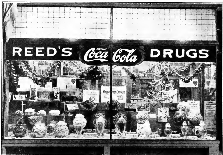
Fig. 21.—Show window of the boxed-in type illuminated with five single inverted mantle gas lamps installed over glass panels in the ceiling of the window close to the plate glass.
