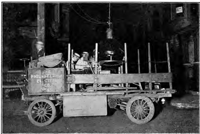
Fig. 33.—Integrating sphere photometer in service tests.
