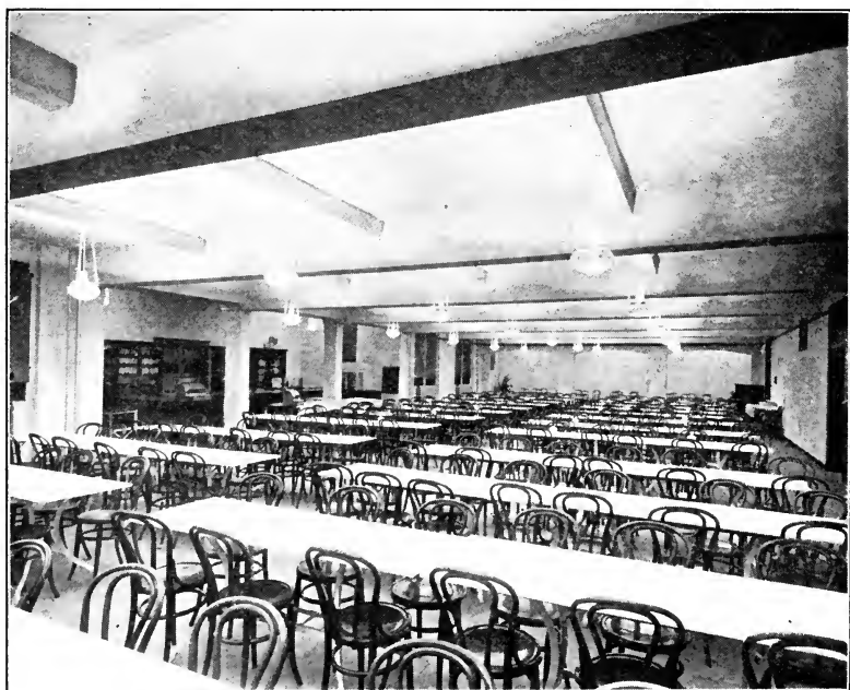
Fig. 12.—Luminous bowl, indirect illumination in school cafeteria.
