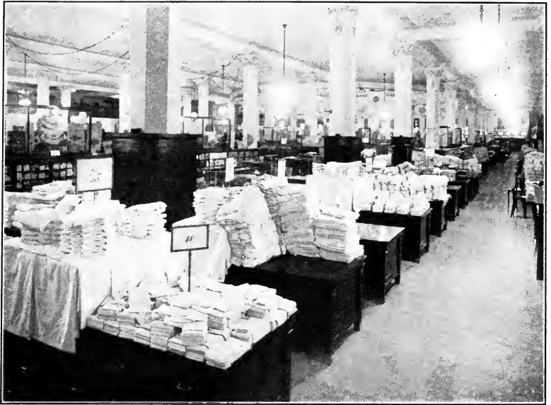
Fig. 7.—Department store floor using single-chain fixtures with one-piece opalescent glass-ball globes. This is a typical department store floor.
