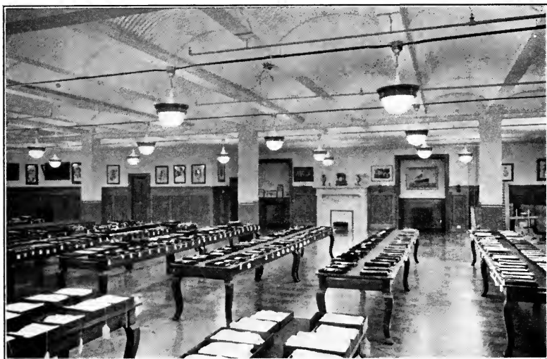
Fig. 4.—Sales floor of large wholesale dry-goods house using a form of semi-indirect fixture with translucent bowl and wide band, the interior of which is lined with ripple mirrored glass. 250-watt vacuum tungsten lamps were used, one at each outlet, with a spacing of 11 ft. by 15 ft. On this floor the ceiling and upper side walls are finished in a flat white.
