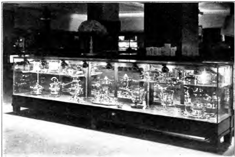
Fig. 13.—Show case lighted with small individual reflectors using 15-watt round bulb candelabra base tungsten lamps. These reflectors are usually installed on 10-in. to 24-in. centers. The reflector equipment is also adapted to small lamps and medium screw-base receptacles.
