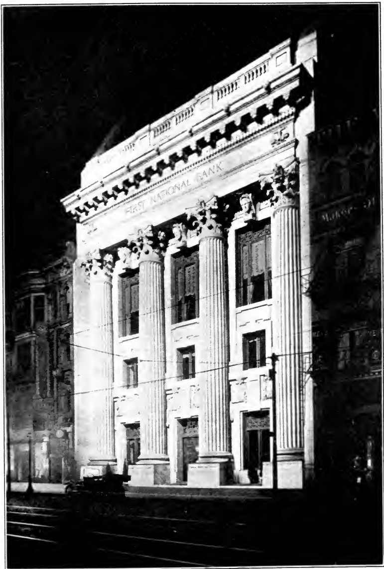
Fig. 30.—Representative flood-lighting installation.
