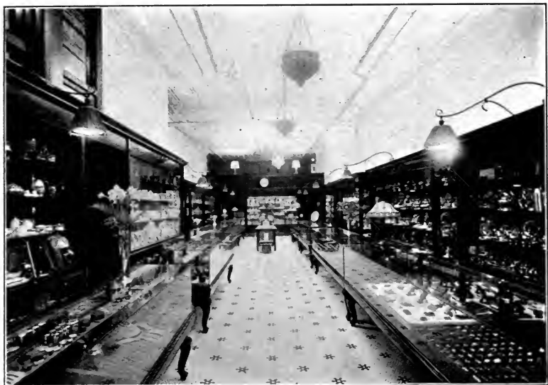
Fig. 5.—General view of jewelry store lighted with indirect lighting fixtures for general illumination and direct lighting units bracketed out from the shelving over the counters. Store 22 ft. by 60 ft., ceiling height 16 ft. Length of fixtures 3.5 ft., using in the five outlets three 500-watt lamps and two 750-watt lamps, the latter on outlets No. 2 and 4.
