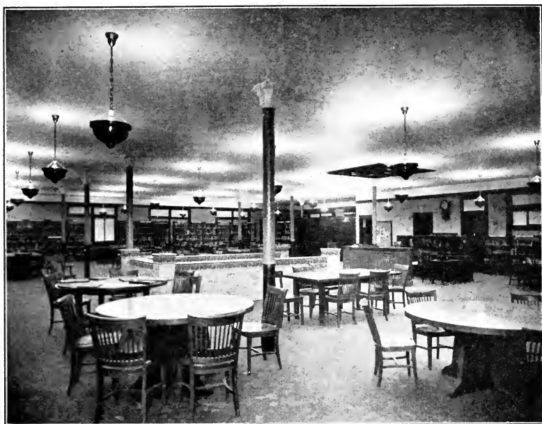
Fig. 19.—Indirect illumination in a branch library in a large city.
