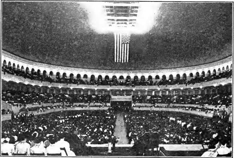
Fig. 36 —Glaring lamps in auditorium lighting.
