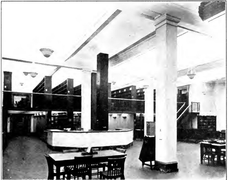
Fig. 14.—Reading room and book stacks illuminated entirely by indirect-lighting units.
