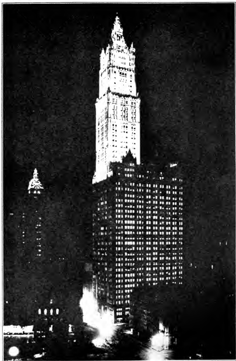
Fig. 32.—Representative flood-lighting installation.
