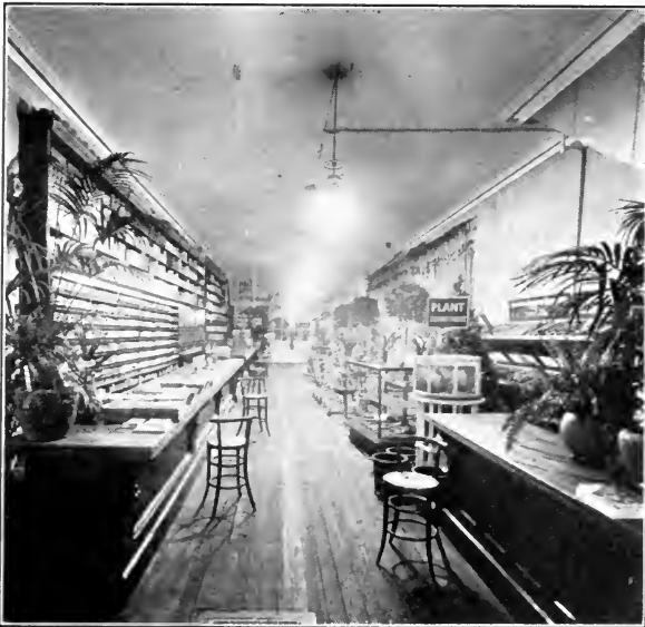
Fig. 10.—A plant and seed store using inverted mantle "gas arc" lamps. This type of installation is favored in those places where low first cost is the most important consideration.
