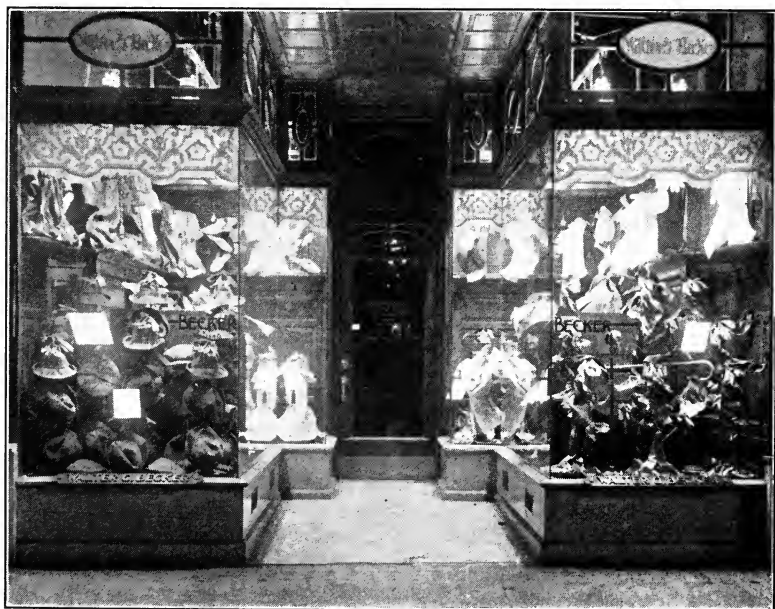
Fig. 22.—A deep enclosed window with glass panels in the ceiling above which gas lamps with concentrating reflectors are used.
