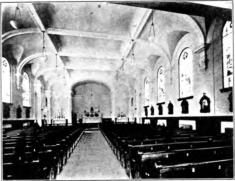
Fig. 9.—Ritualistic church. Semi-indirect lighting; two rows of fixtures. Concealed lighting back of sanctuary arch.
