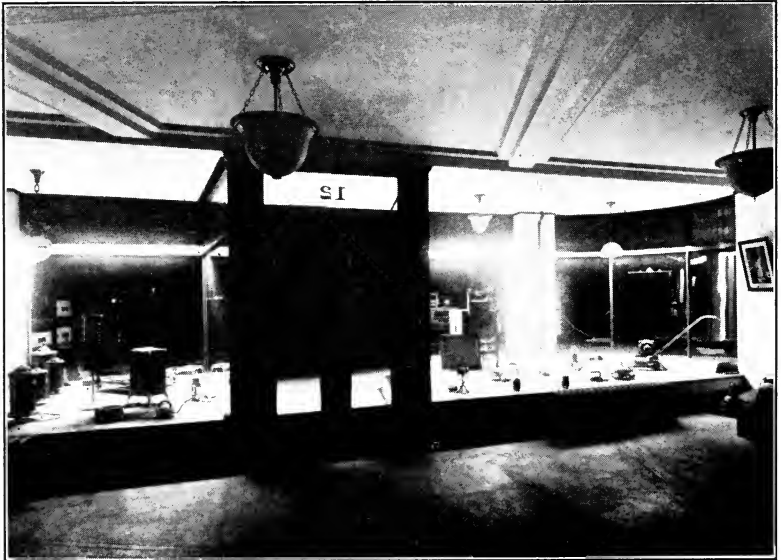
Fig. 16.—Show window, open in the back. Lamps in trough reflector screened from the view of those in the interior.
