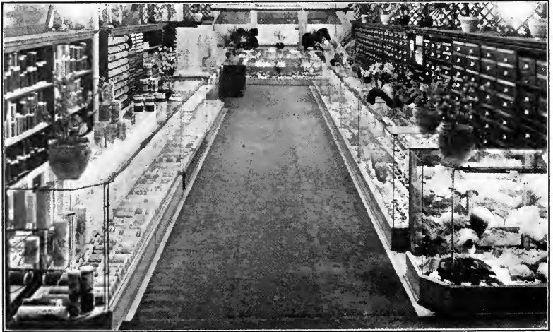
Fig. 12.—Show cases with small continuous trough reflectors using 11 in. tubular lamps with single straight filament and contacts on each end of the tube. This equipment for case lighting occupies a minimum of space in the corner of the case and is reasonably inconspicuous.
