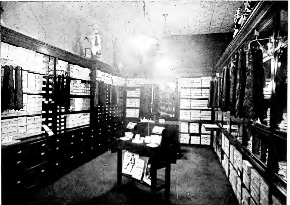
Fig. 7.—A small haberdashery shop (30 x 15 feet) lit by three 200-watt Mazda C Daylight lamps in enclosing, light directing, luminaires. The ten foot-candles of general illumination enables one to make critical selection of the merchandise on display.
