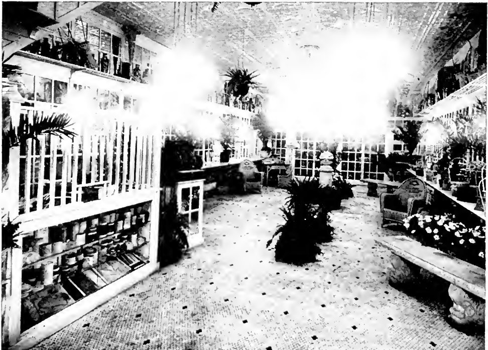
Fig. 11.—Light is a valuable decorative medium in the florist shop. This establishment (50 x 20 feet) is carefully planned, well painted and maintained. It is lighted by seven multiple unit luminaires, each supplying five 40-watt Mazda B lamps in spherical opalescent diffusing globes. The average intensity is in the neighborhood of eight foot-candles. It is a pleasure to shop amid such surroundings.
