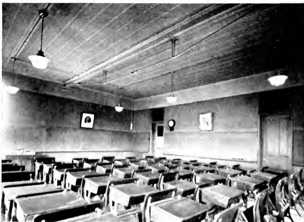
Fig. 7.—Outhwaite School, day view of typical test installation, six-unit lay-out, squat shape, opalescent glass enclosing globes.
