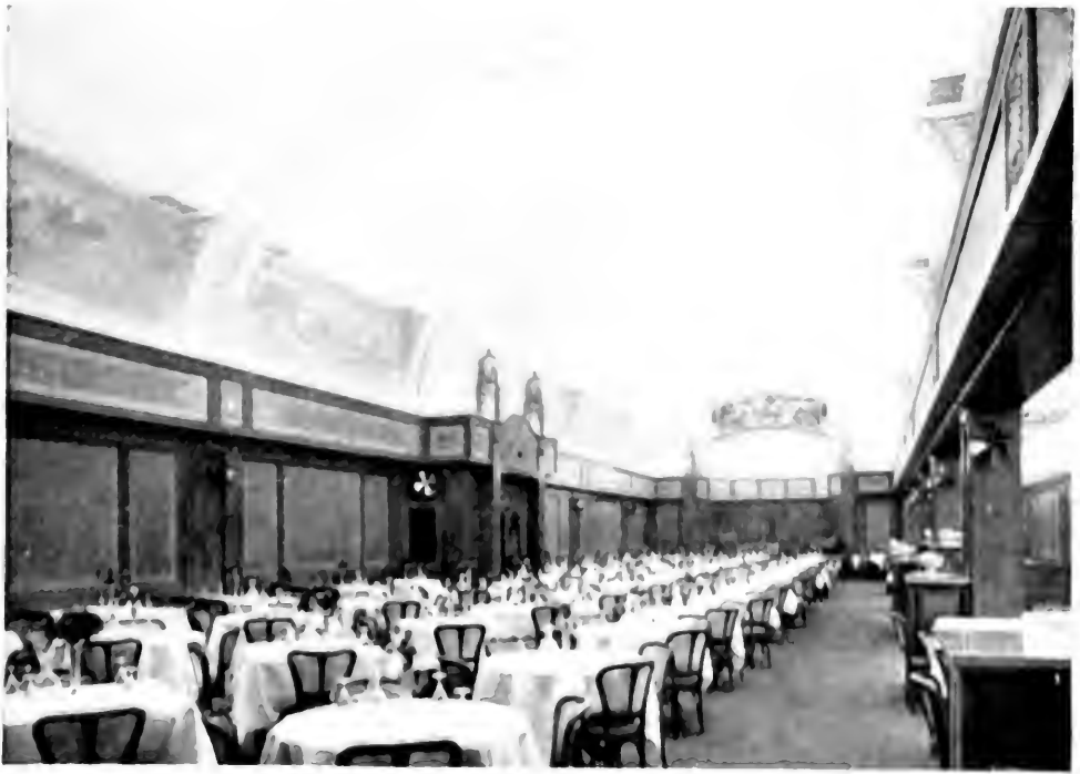
Fig. 18. Public restaurant in which cove lighting method was employed with success.
