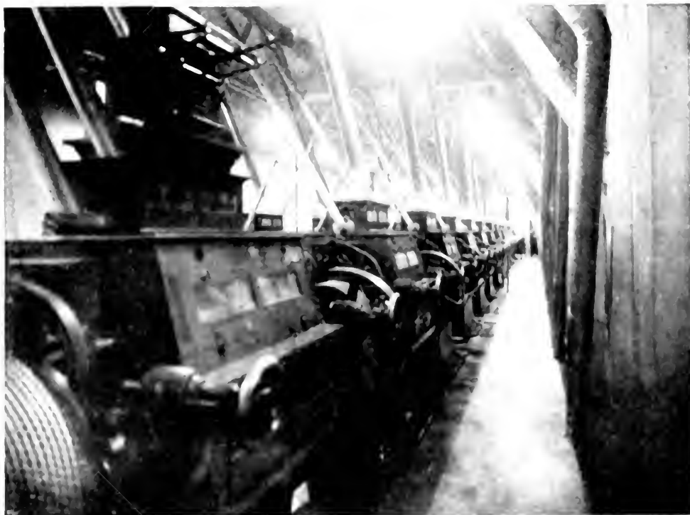
Fig. 6. High level lighting of the roller floor in a progressive flour mill. 150 watt bowl enameled Mazda C lamps in R1.M standard dome reflectors are 10 feet above the floor on centers 8 x 10 ft, the intensity is over 12 ft.c.
