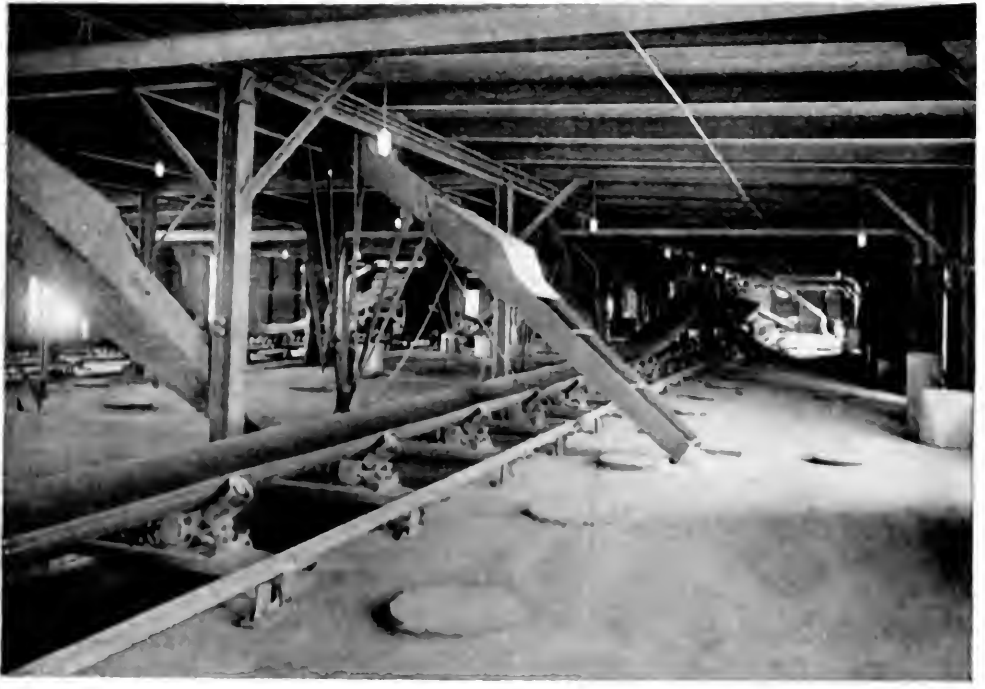
Fig. 2.—Day view illustrating typical conditions encountered in a grain elevator, 25 watt Mazda B lamps in vapor proof globes on centers 12 x 14 feet. Absence of reflectors and dust accumulation results in decidedly low utilization of light, average intensity less than 0.5 ft.c. Inadequate as it may seem it pictures one of the best installations inspected.
