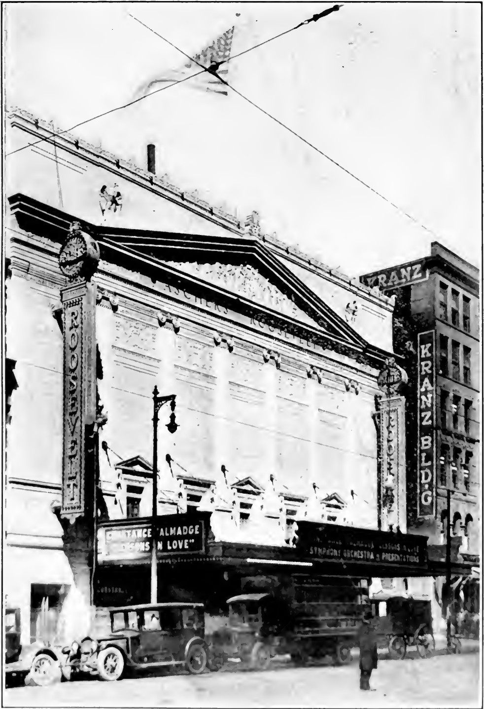
Fig. 5.—The signs carry out the architecture of the building and by the use of castings and ornamented supports are made to be just as attractive as the fine building front. The architect was Mr. C. Howard Crane of Detroit, Mich., for this and the Music Box Theatre.
