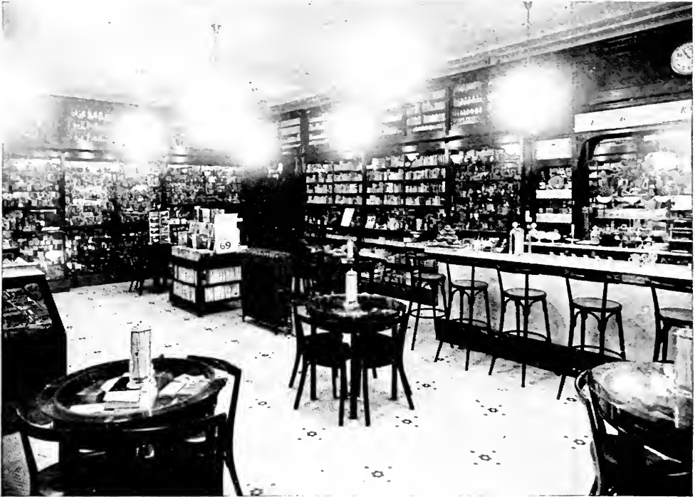
Fig. 10.—A modern drug store (40 x 30 feet) as it appears by night, lighted by twelve 200-watt Mazda C lamps in light directing enclosing luminaires. This merchant believes in the drawing power of light, and provides eleven foot-candles of general illumination.
