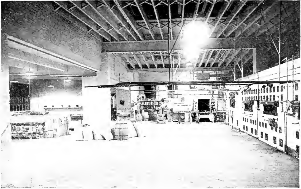
Fig. 7.—A rare example of modern lighting applied to the mixing and bake room of a progressive medium sized bread bakery. The 18 x 18 feet bays in front of the ovens are illuminated by centrally located 200-watt clear Mazda C lamps in RLM standard dome reflectors producing a resultant intensity of approximately 3.5 ft.-c.
