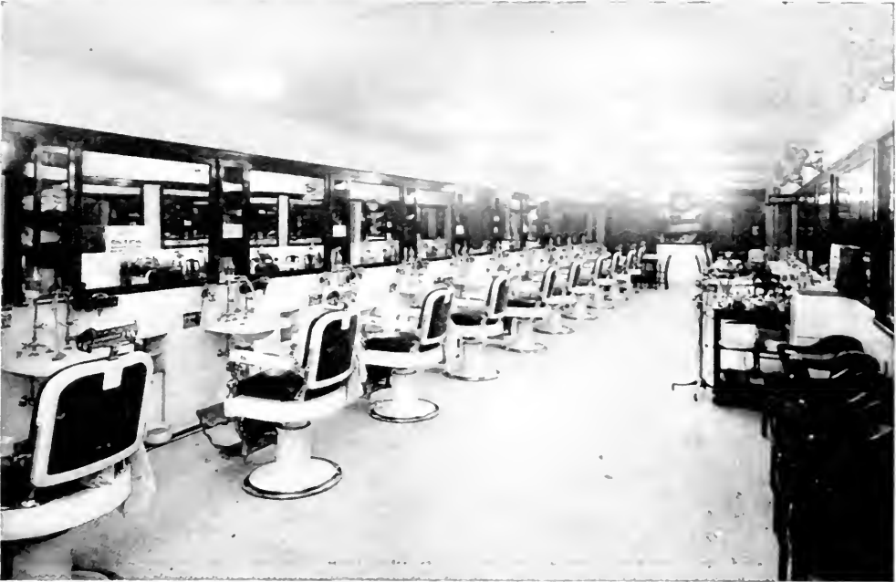
Fig. 4.—A thoroughly up to date barber shop (70 x 15 feet) illuminated by fourteen 100-watt Mazda C lamps in enclosing semi-indirect luminaires. These are placed close to the ten foot ceiling. A uniform intensity of over five foot-candles prevails.
