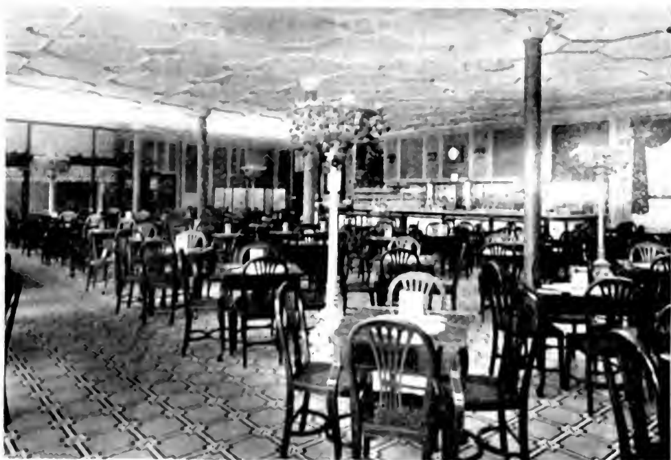
Fig. 12—The Hopper. A tea room lighted in an unusual manner.
