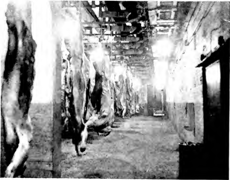
Fig. 10. Night view of a typical "Sales Cooler" illuminated by 60-watt bare Mazda B lamps on center, 8 x 6 feet producing an average intensity of 8 ft.c. The light surroundings and in the utilization of light and minimization of glare from the unshielded lamps.
