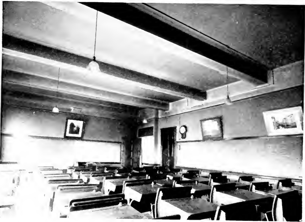
Fig. 2.—Outhwaite School, Cleveland, day view of original installation, four 100-watt bowl frosted Mazda C lamps in prismatic glass, direct lighting reflectors.
