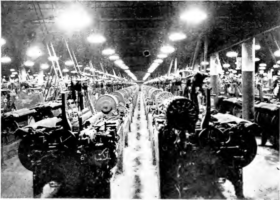
Fig. 8.—This denim weave room uses one 75-watt lamp in an R.I.M. dome for each loom.
