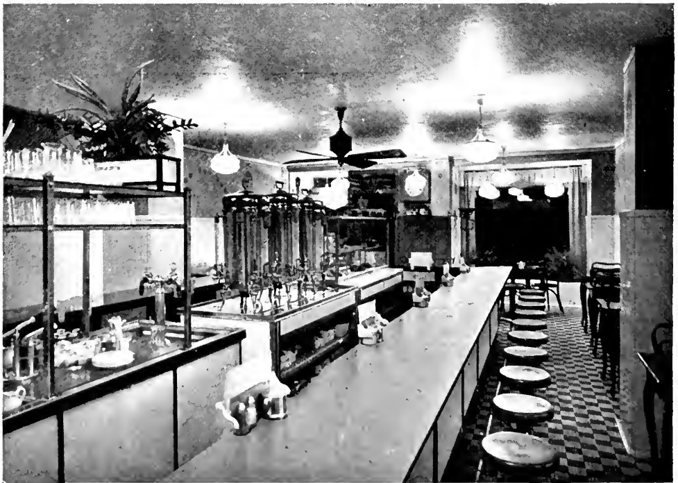
Fig. 5. Interior typical of the commercial restaurant. The low ceilinged room, in which the luminous type of indirect fixture is suspended on short chains, gives excellent lighting results.
