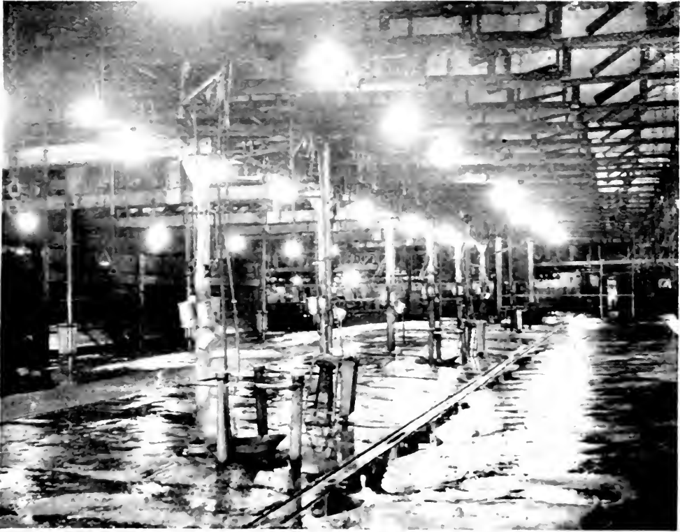
Fig. 9. A night view of the killing and stripping floor of a modern packing plant. 150-watt bowl-enamelled Mazda C lamps in shallow dome porcelain reflectors on 10-foot centers, assisted by light-colored surroundings, furnish a well-diffused illumination of approximately 12 ft.c. intensity.
