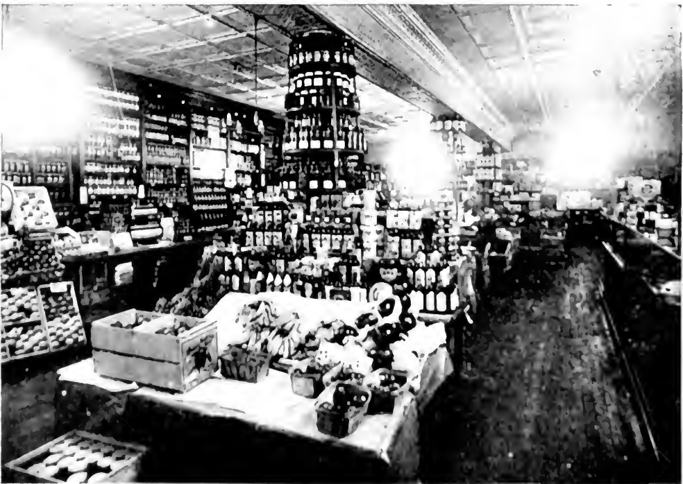
Fig. 7.- Night view of a progressive grocery store (100 x 100 ft.) lighted by eight 100-watt and four 200-watt Mazda C lamps in a new and attractive design of opalescent enclosing globe. Although outlets are spaced only 10 ft. centers, the illumination is in the order of 18 foot-candles throughout the store.
