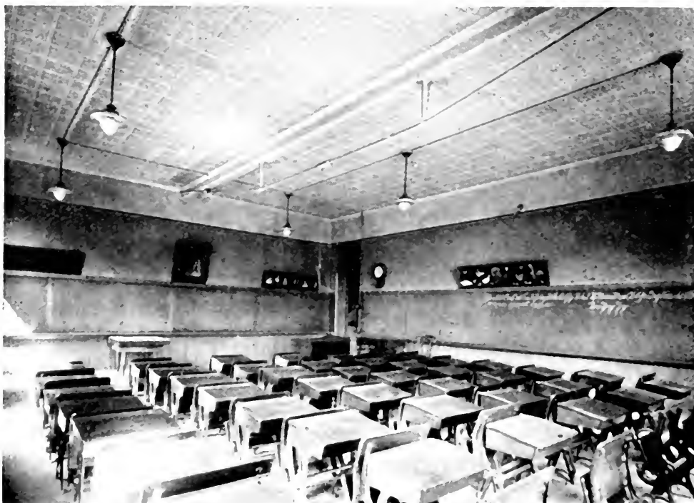
Fig. 6.—Outhwaite School, day view of typical test installation, six-unit lay-out, enamelled and crystal glass enclosing direct lighting globes.
