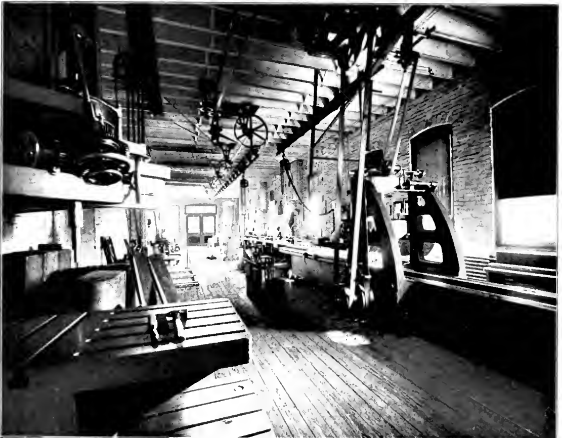
CORNER IN MACHINE SHOP—SHOWING LARGE RADIAL DRILL AND HEAVY PLANER.
