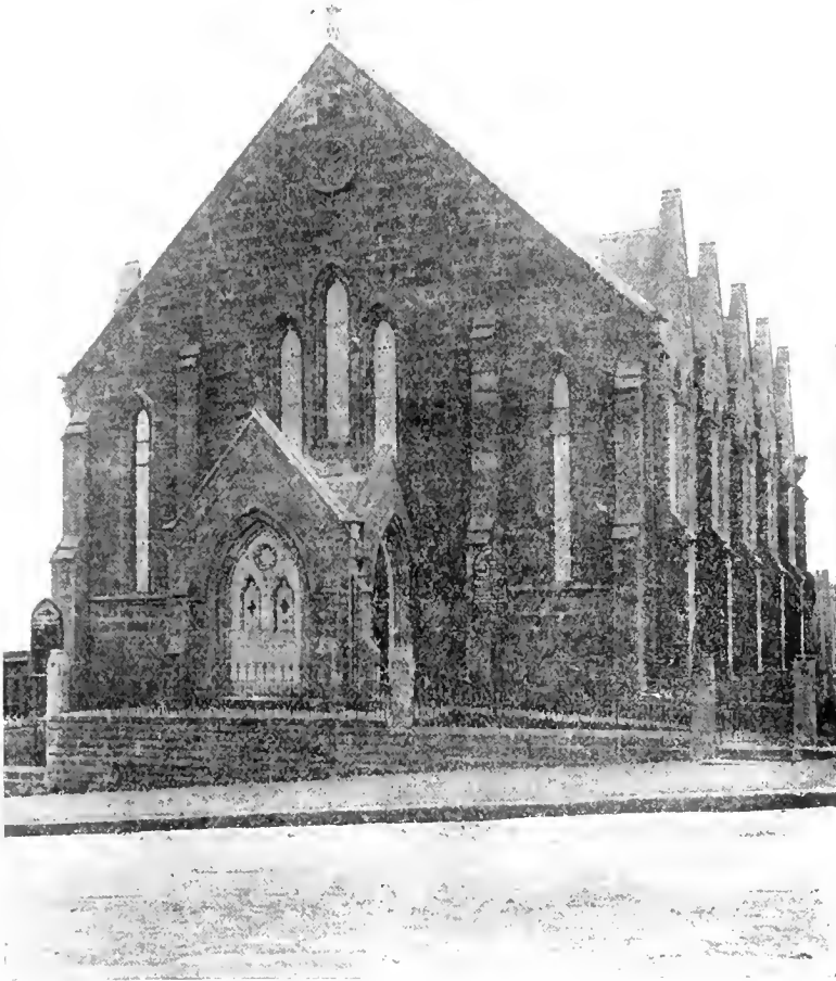
DARLING STREET CHURCH, BALMAIN.
