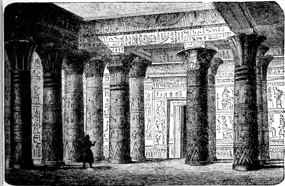
PILLARED HALL FROM THE TEMPLE AT PHILÆ IN EGYPT.
