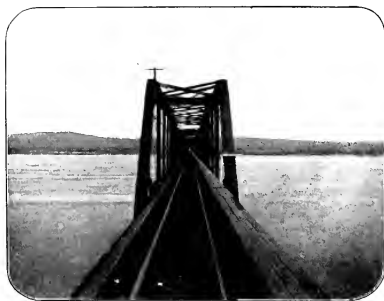
RAILROAD BRIDGE ACROSS THE COLUMBIA AT KENNEWICK
