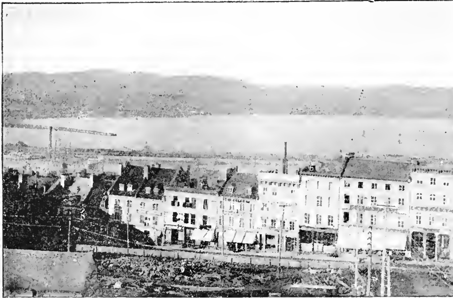
FABRIQUE STREET, LOOKING TOWARD BEAUPORT.
