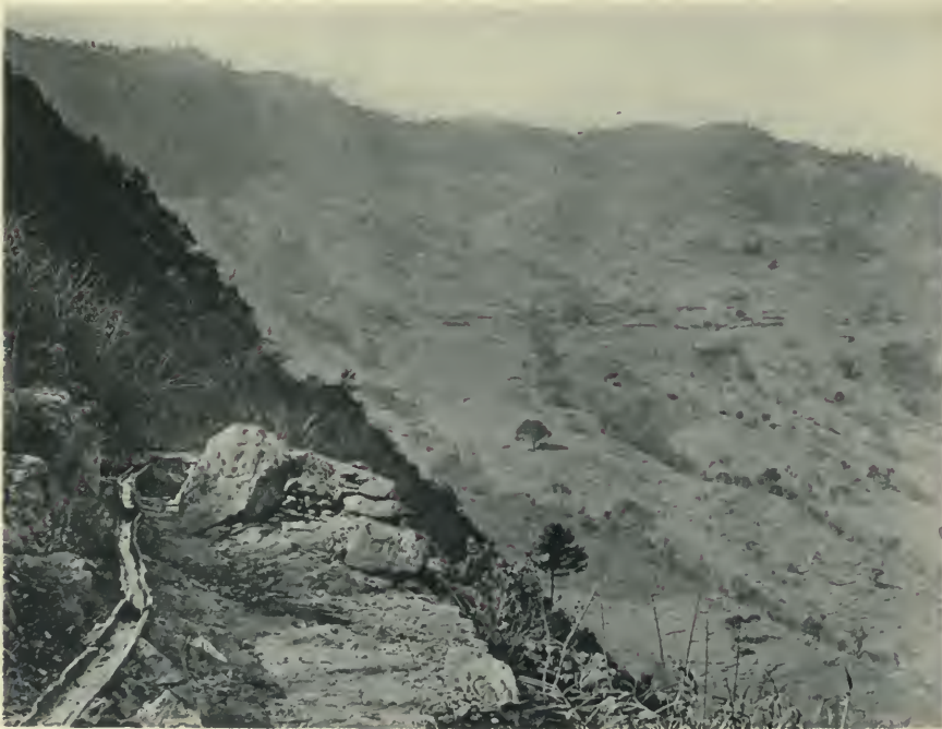
OLD FALAM : WHERE PERMANENT POST WAS BUILT.
