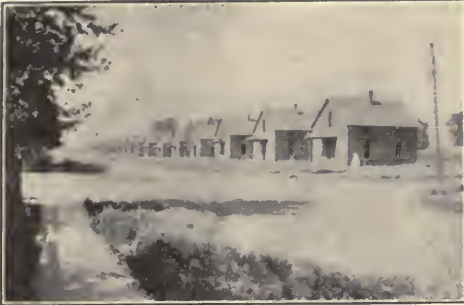
No housing shortage here. A row of 20 houses in Cherry, only 2 of which were occupied in August, 1920.
