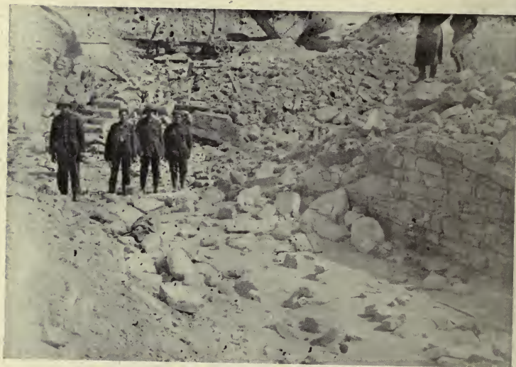
1. EXTERIOR OF SEDD-UL-BAHR FORT.
