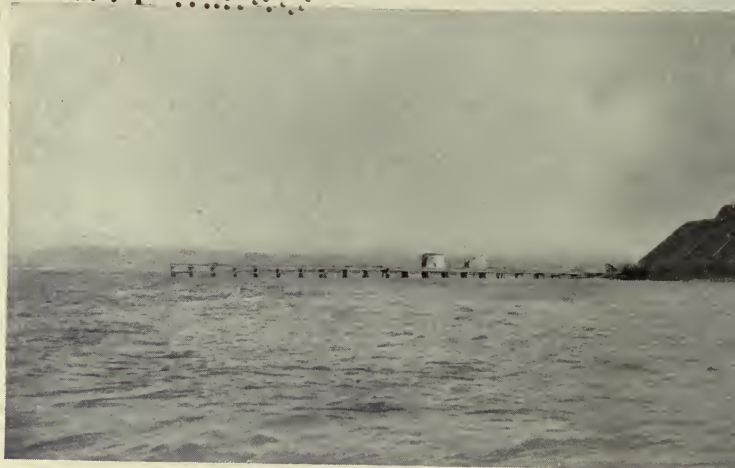
FORT 6, KUM KALE, TO WHICH A TOW OF BOATS WAS BEING
