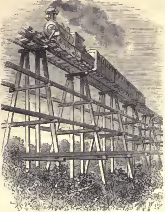
Trestle-work Viaduct, United States.
