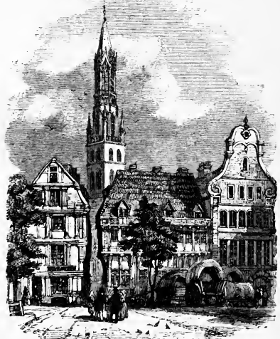
TOWER OF THE CHURCH OF ST. JAMES, AND HOUSES OF THE 16TH AND 17TH CENTURIES, HAMBURG — From Dendoff.
