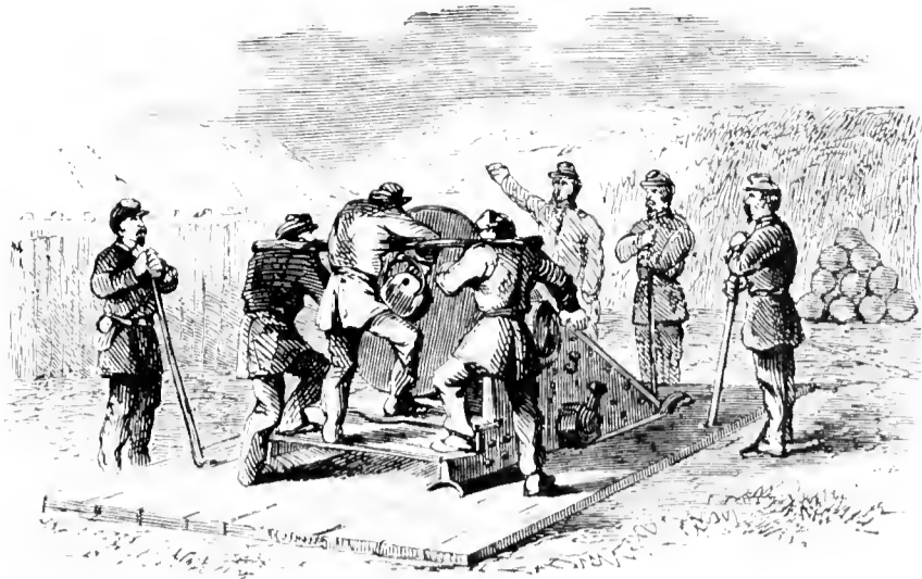
MORTAR PRACTICE—PUTTING IN THE SHELL.
