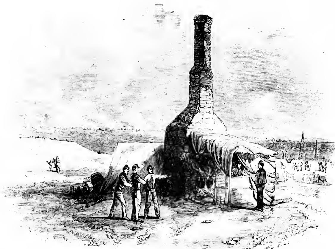
ARMY COOKHOUSE CONSTRUCTED IN AN OLD CHIMNEY OF AN OUTHOUSE OF THE LACY MANSION, ON THE RAPPAHANNOCK, FALMOUTH, VA.
