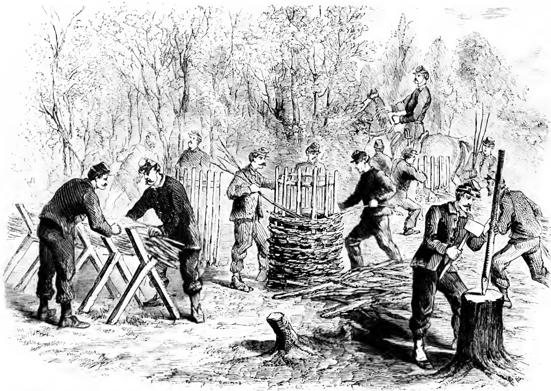
CAPTAIN MULLER'S BATTERY COMPANY OF THE SEVENTY-SEVENTH PENNSYLVANIA REGIMENT MAKING FASCINES AND GABIONS FOR BREASTWORKS.
