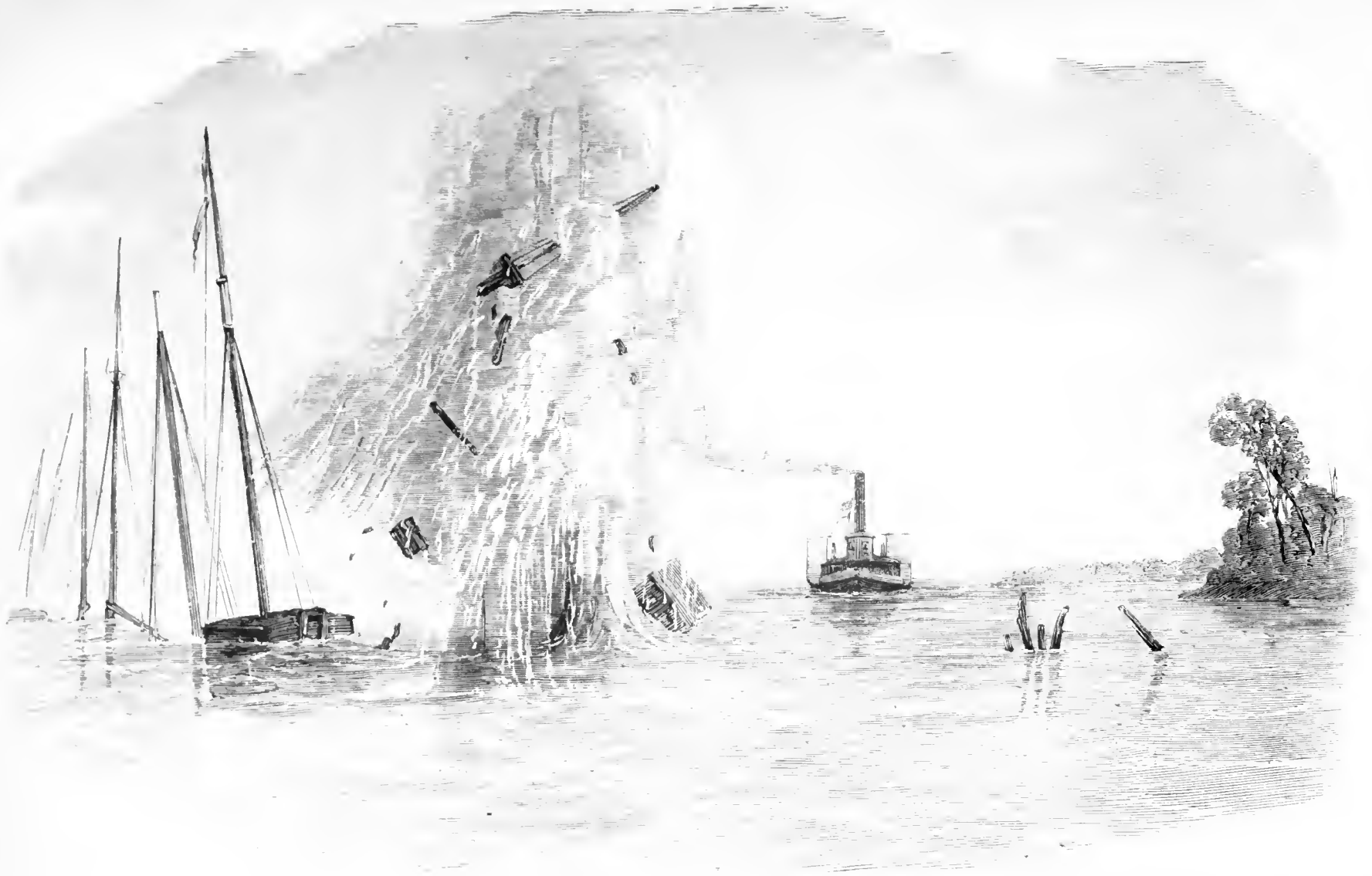
REMOVING SUNKEN SCHOONERS FROM CORE SOUND, N. C., PLACED TO OBSTRUCT THE PASSAGE OF THE FEDERAL GUNBOATS, UNDER THE SUPERINTENDENCE OF CAPTAIN HAYDEN, OF THE NEW YORK SUBMARINE ENGINEERING COMPANY.
