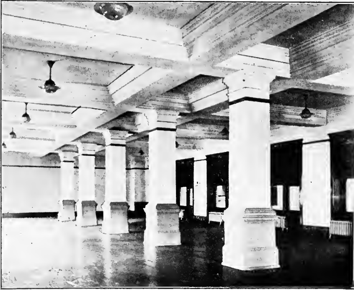
9.—EAST ROOM ON THE SECOND FLOOR OF THE VERMONT BUILDING.
