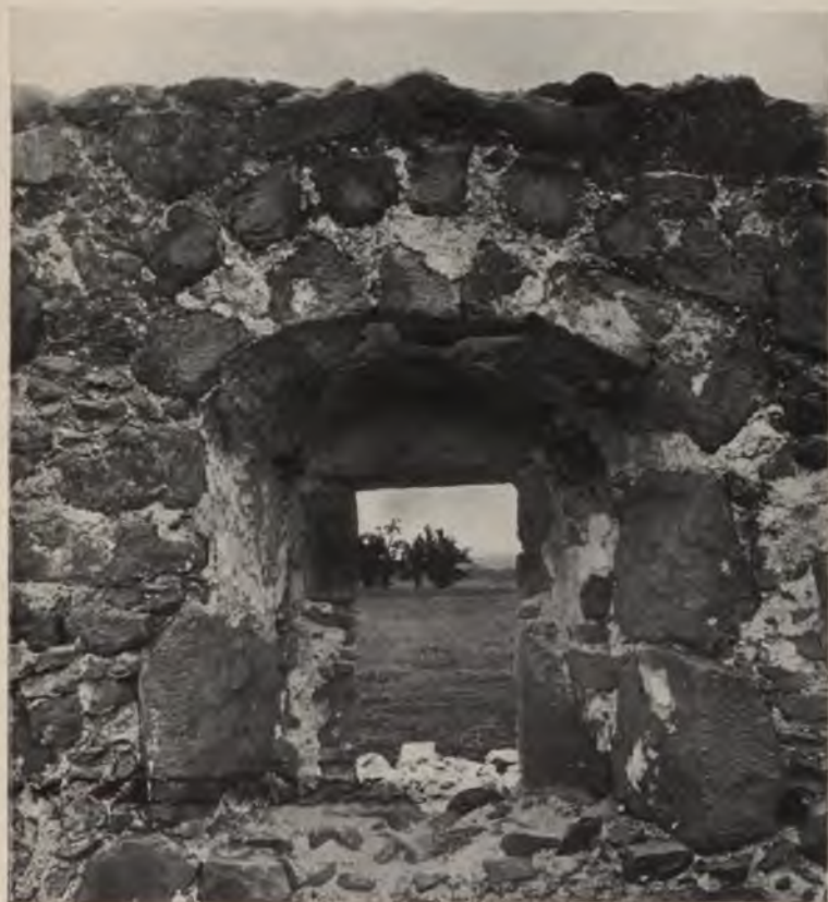
STONE ARCHED DOORWAY, SANTA MARGARITA CHAPEL
