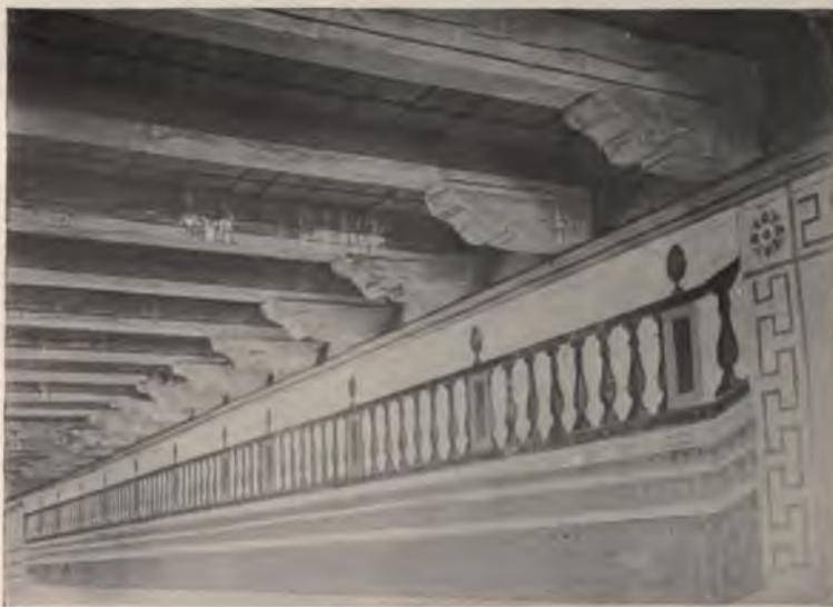
b. CORBELS AND RAFTERS OF SAN MIGUEL MISSION
