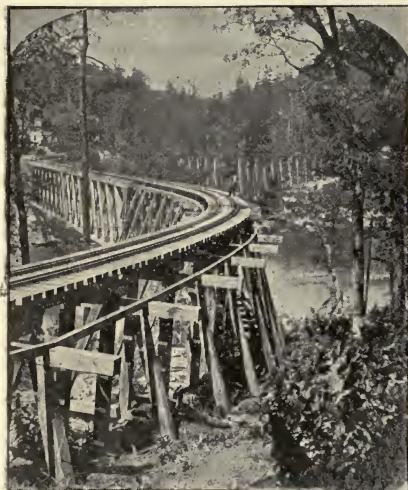
RAILROAD BRIDGE NEAR CLARION.
