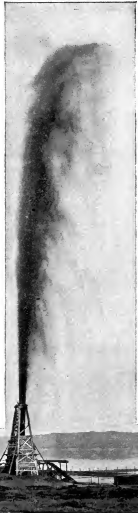
WELL AT BAKU, RUSSIA, FLOWING 50,000 BARRELS A DAY, THROUGH A 16-INCH PIPE.
