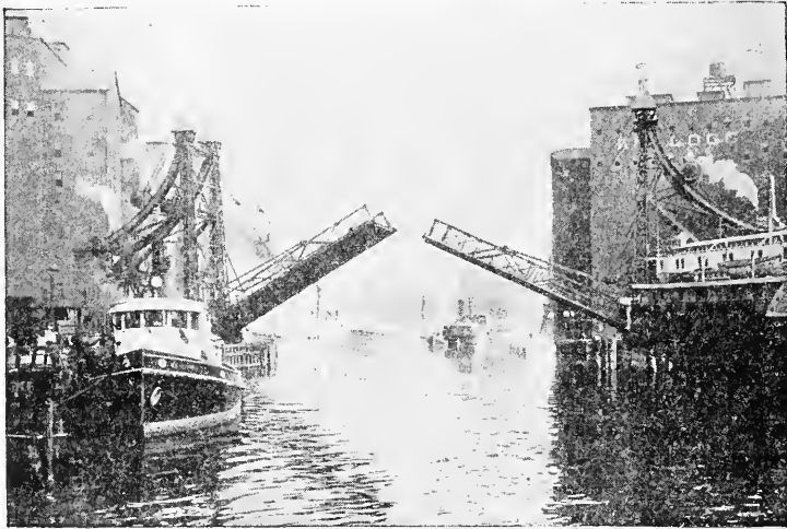
BASCULE BRIDGE AT MICHIGAN STREET
