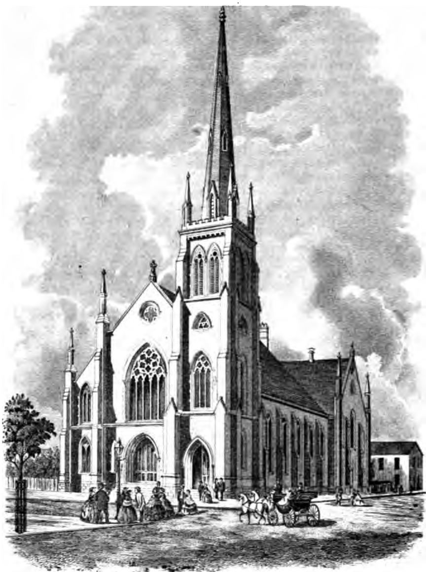
Methodist Episcopal Church INDIANAPOLIS
