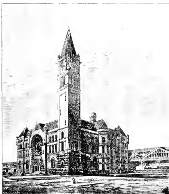
Union Station, Indianapolis.
