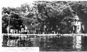
Swimming Pier Completed
