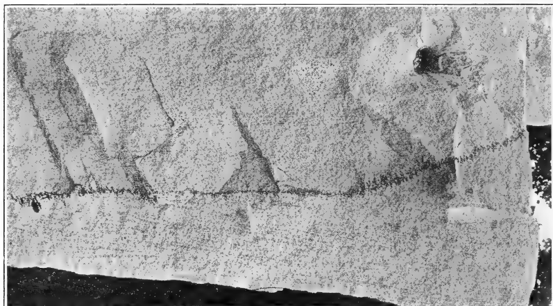
FIG. 17.—Stylolite-seam which leaves the bedding plane and cuts across the lamination of the upper stratum at an angle of about 20 degrees. From a quarry of the Consolidated Stone Company, Hunter Valley district, Monroe County, Ind.
