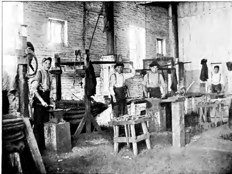
THE BLACKSMITH SHOP INTERIOR
