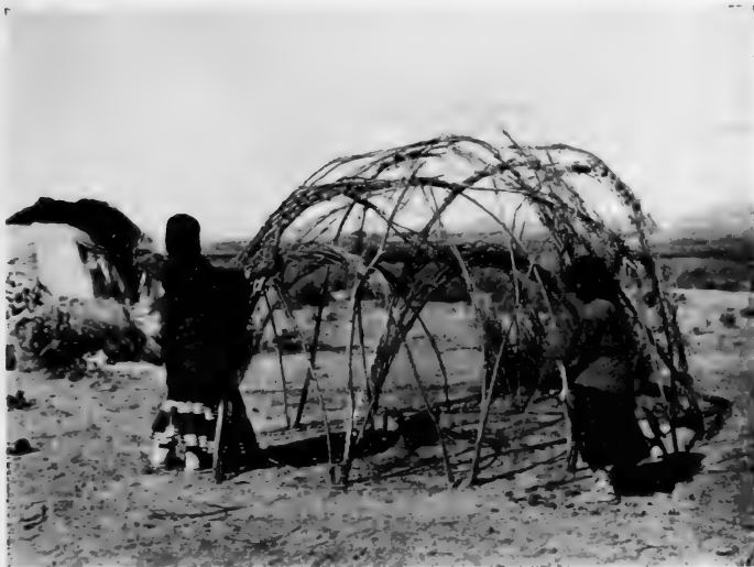
San Carlos Apache Women building a House
