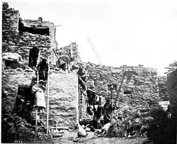
HOPI WOMEN BUILDING A HOUSE AT ORAIBI.
