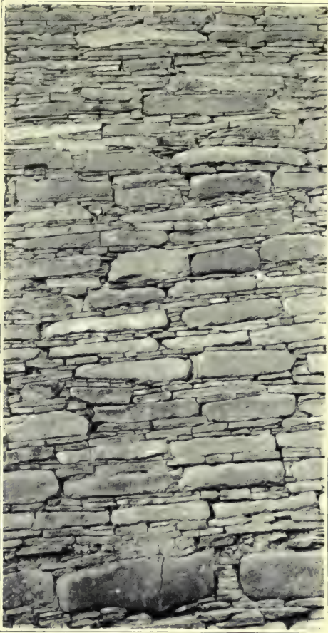
Portion of Masonry Wall. Chaco Canyon. (Courtesy of Dr. Prudden.)
